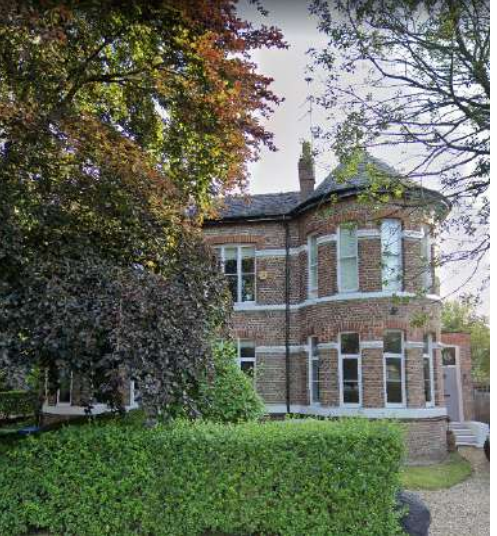
Neighbouring Villa with rotunda feature
