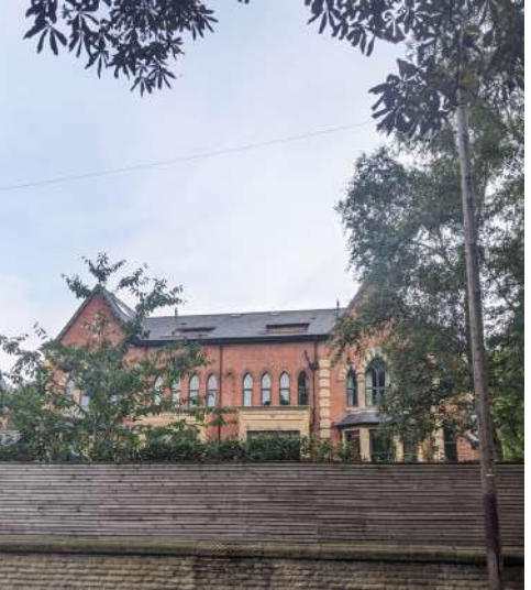
Westbrook Villas (Edge Lane)
