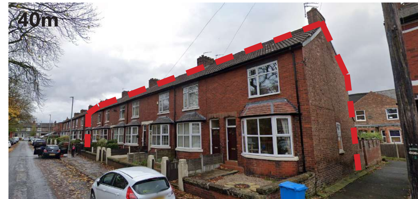
Demonstrating the approximate length of surrounding residential buildings
