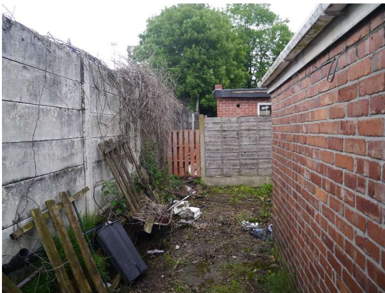
Gable boundary to adjacent Industrial Site.
