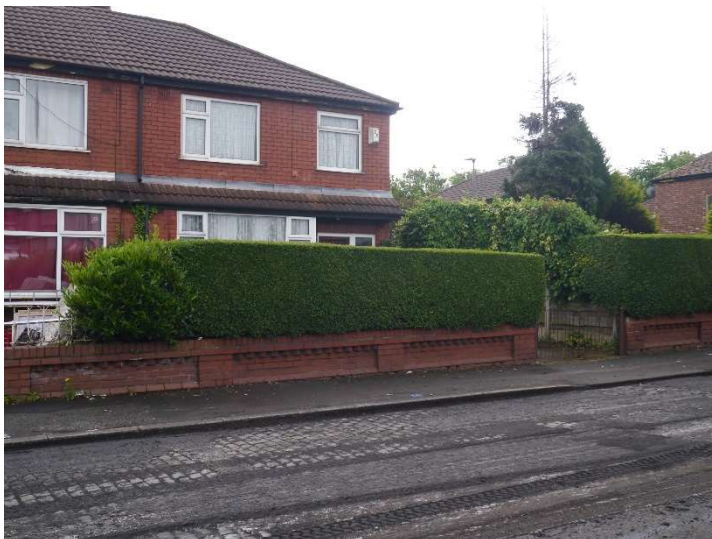
Front Elevation of adjacent property. Nr 301
