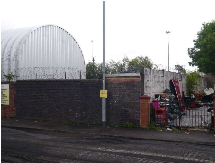
Industrial site adjacent to application property.
