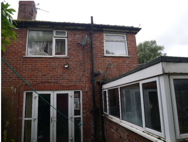
Rear Elevation of application property.
