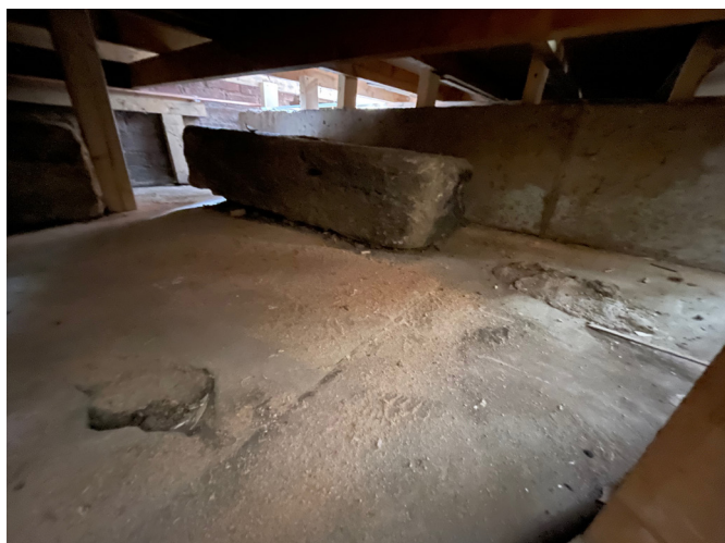
Image 7: Photograph of underside of internal deck showing modern concrete, supporting the external deck, which was added in 1994.
