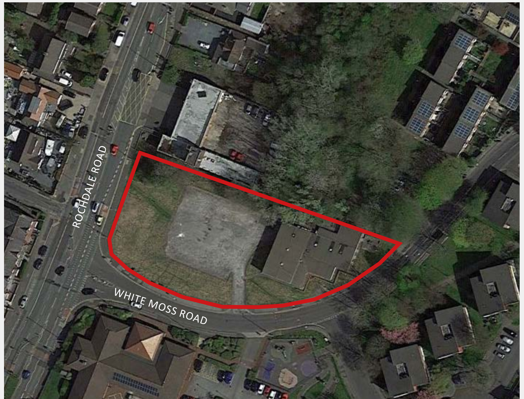
— Aerial View of Site
