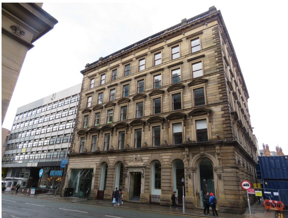
Figure 1: Principal elevation to 37 Peter Street / Freetrade Exchange from Peter Street.
