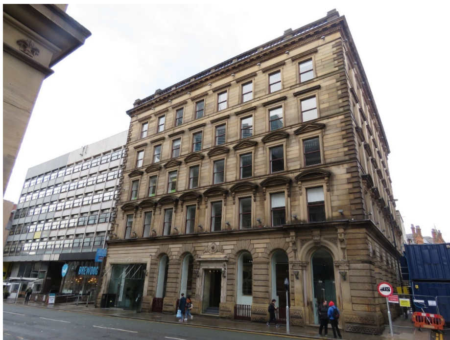
Figure 12: 2021 – Image of the Site as known as ‘Freetrade Exchange’, looking north from the south side of Peter Street. The adjacent 35 Peter Street now demolished and replaced in the 1960s with the office building that survives today. The building underwent a comprehensive refurbishment in 2007 following the grant of planning permission in 2004. The development re-branded the building from Harvester House to Freetrade Exchange.
