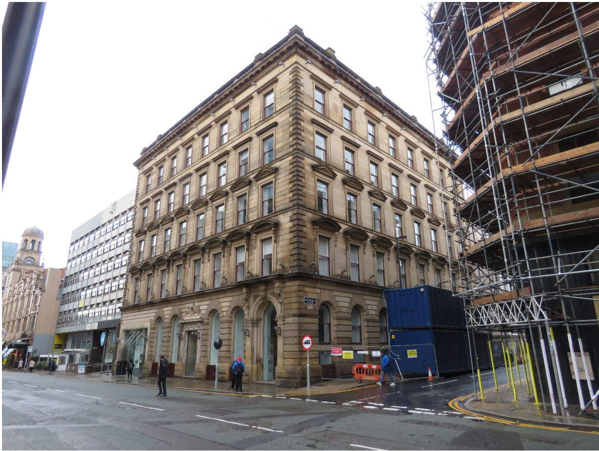
Figure 15 – View along Peter Street looking west with 37 on the right hand side and the Freetrade Hall on the left, opposite on the intersection also sits 47 Peter Street and the Theatre Royal.
