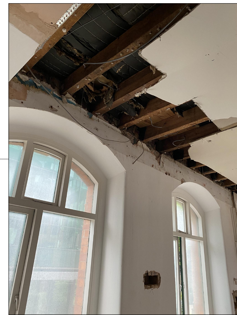
IMAGE 3 Existing ceiling soffit with exposed sections of timber joists to be underdrawn and made good with MF plasterboard
