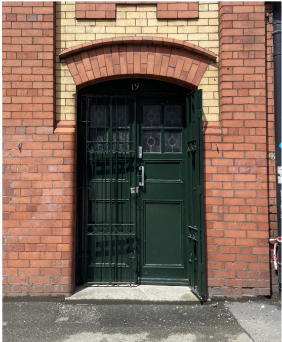
existing side entrance to 19 Mason St
