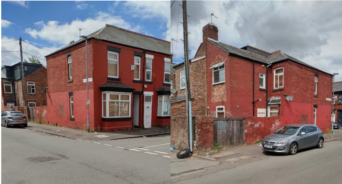
Fig. 1 – Front and rear of 72 Braemar Road
