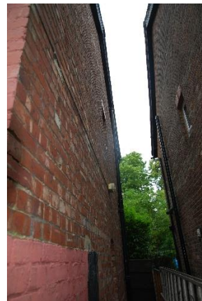
The gable elevation Brickwork with isolated painted areas
