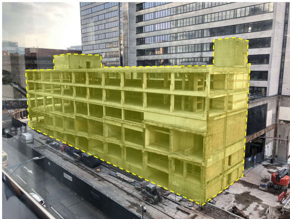
Residual Premier House concrete structure to be removed
