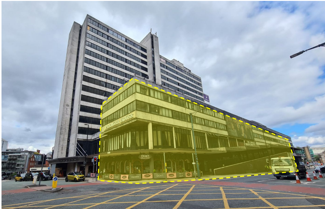
Previous view of Premier House prior to Part Demolition
