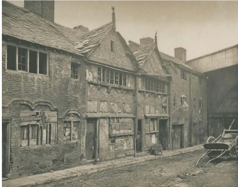
Figure 2: Gibraltar, off Long Millgate in 1877: A group of houses which stood on the banks of the Irk, near Scotland Bridge in a court off the lower end of Long Millgate. A date of 1668 was found on a beam; demolished in 1889. Manchester City Council – Local Image Collection (m80003)
