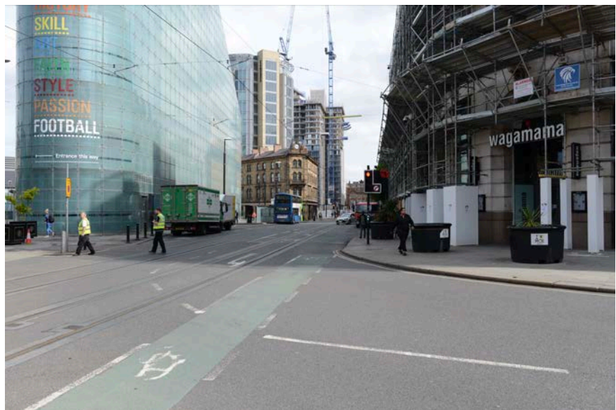
Existing View VP04 : looking north along Corporation Street
