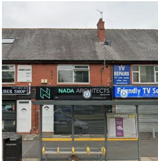
Figure 1 Street view of site
