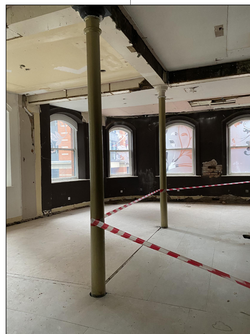
IMAGE 4 Existing historic columns to be left exposed, treated and repainted
