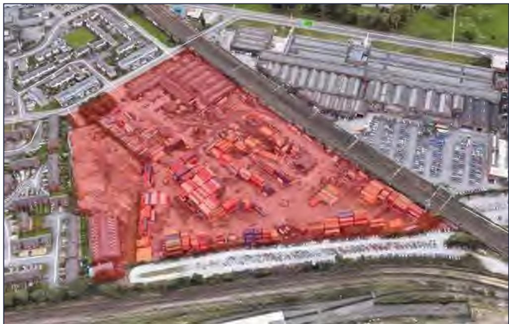
Figure 2.1 – Existing Site and Buildings
