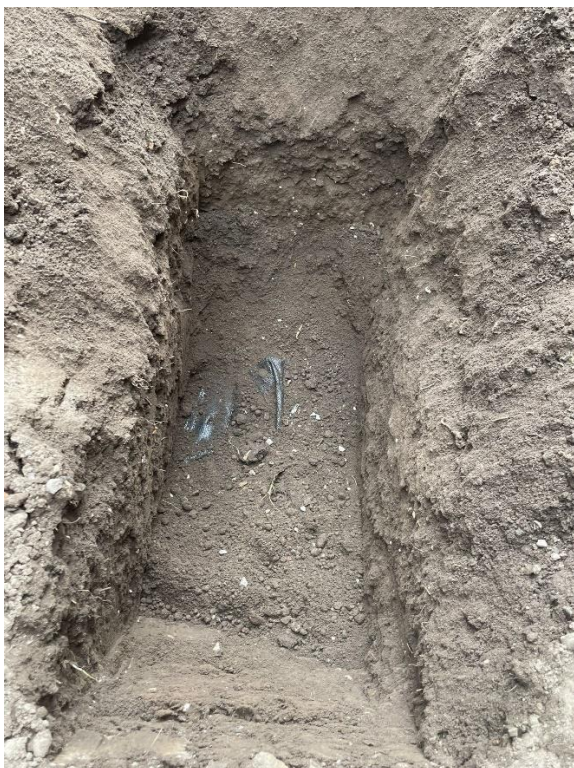
House 1 – 600mm cover system with geotextile membrane
