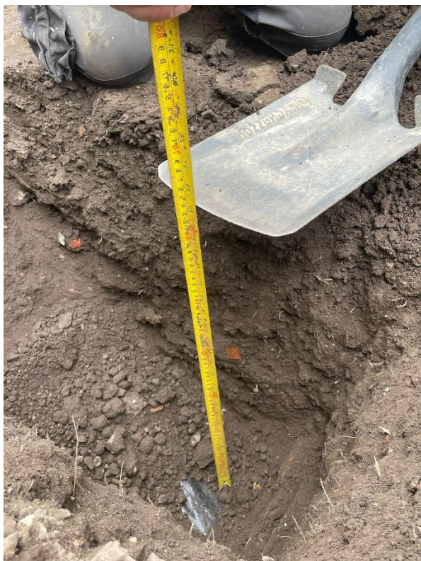
House 4 - 600mm cover system with geotextile membrane
