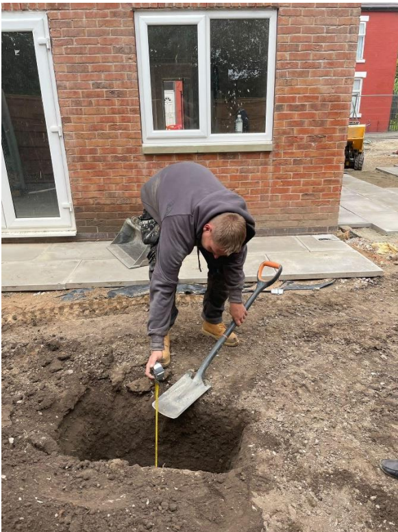
House 2 - 600mm cover system with geotextile membrane
