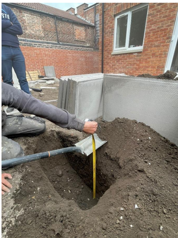
House 4 - 600mm cover system with geotextile membrane
