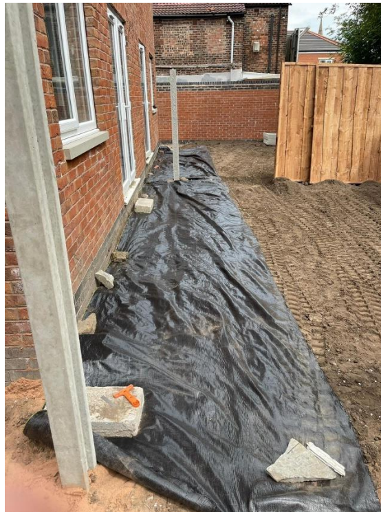
Geotextile membrane in location of patio areas
