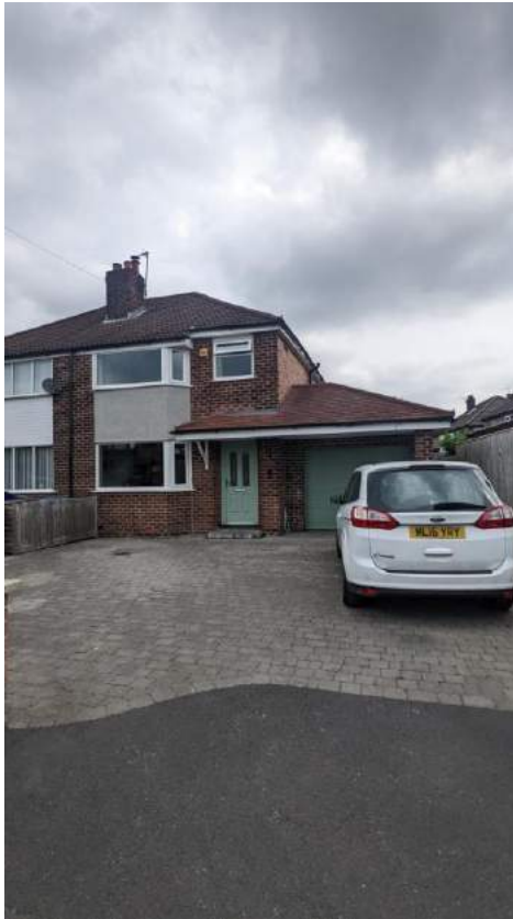
Photo 1 – View of the front of the property
