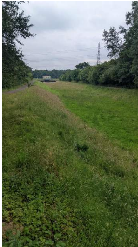
Photo 6 – View of sluice
