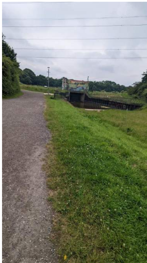
Photo 8 – View of sluice gate
