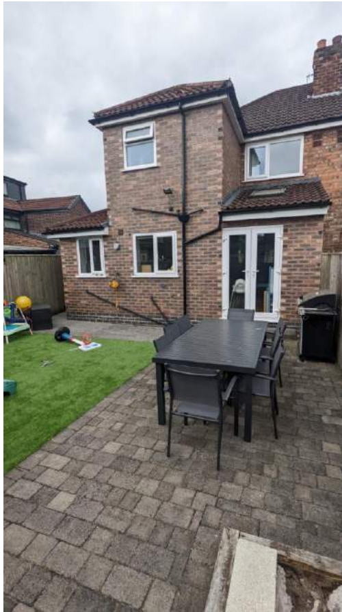
Photo 3 – View at the rear of the property
