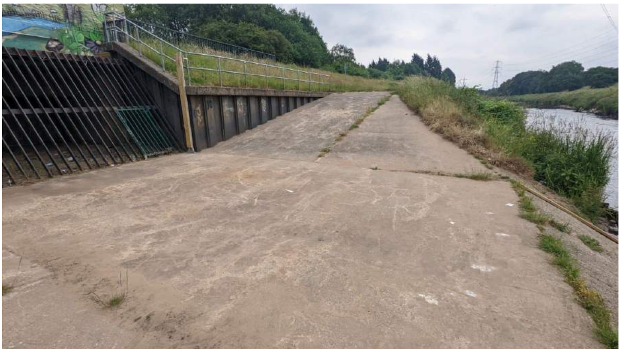
Photo 10 – Debris screen and River Mersey Sluice gate
