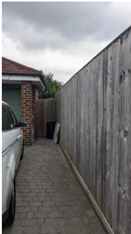
Photo 2 – View of side of the property
