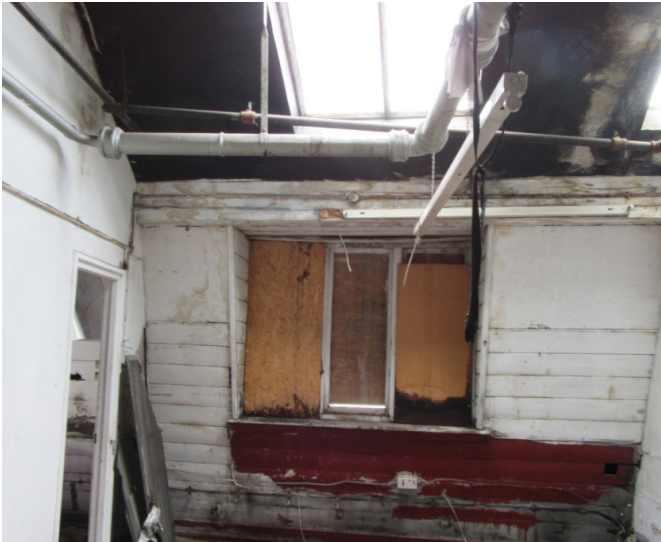
Image 08: The existing non-original windows to fourth floor.
