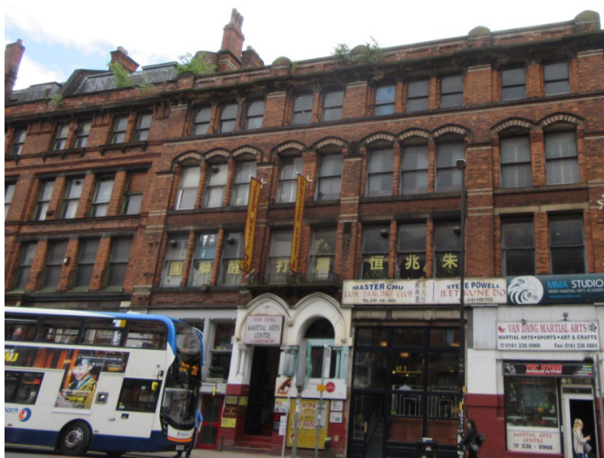
Image 11: External view along Newton Street.
