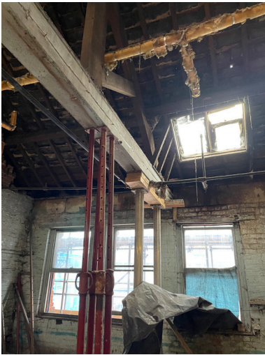
Image 18: Showing ceiling with roof structure exposed.
