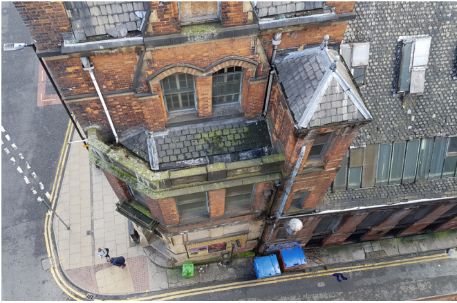
Image 07: Photograph of roof area of second floor; from above.
