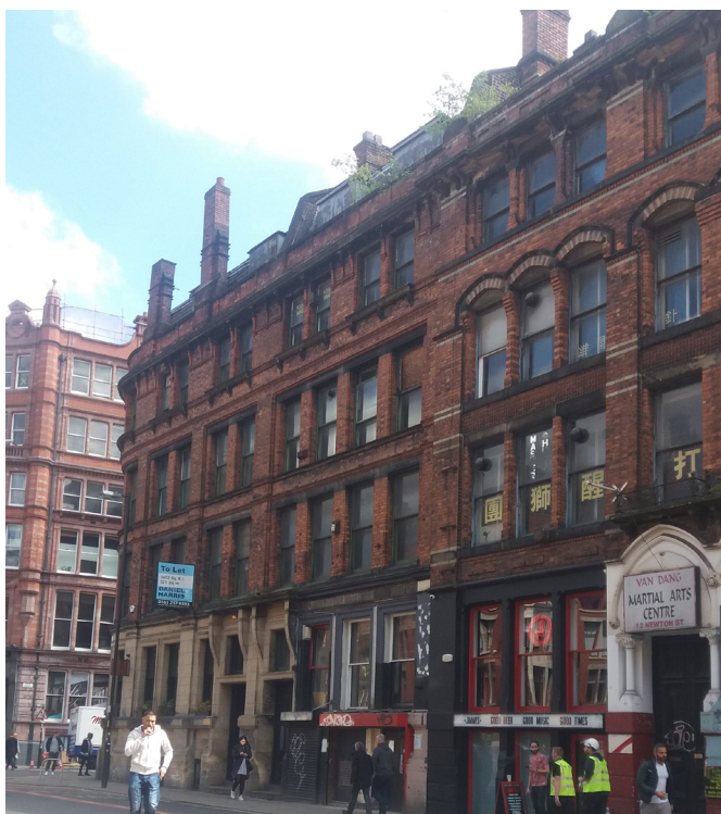
Image 13: View of Newton Street elevation pre-scaffold.
