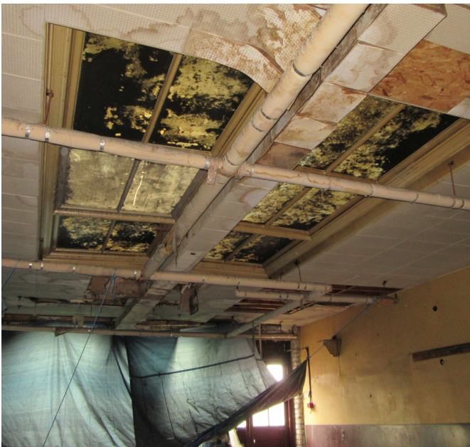
Image 15: Showing non-original ceiling tiles and horizontal windows, taken a number of years ago.
