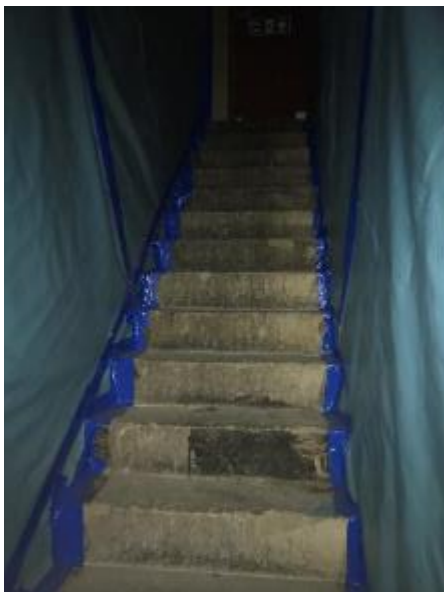
Figure 26: Concrete service stair believed to be contemporary with the original building.
