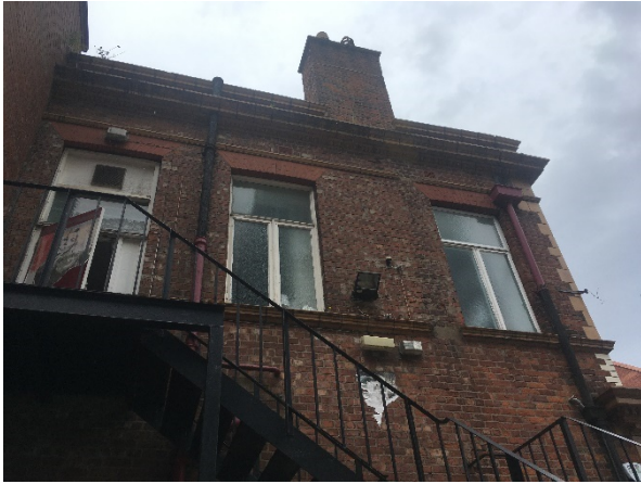
Figure 34: Close up view of the south elevation showing the repaired section of the cornice and gap in the cill string course.
