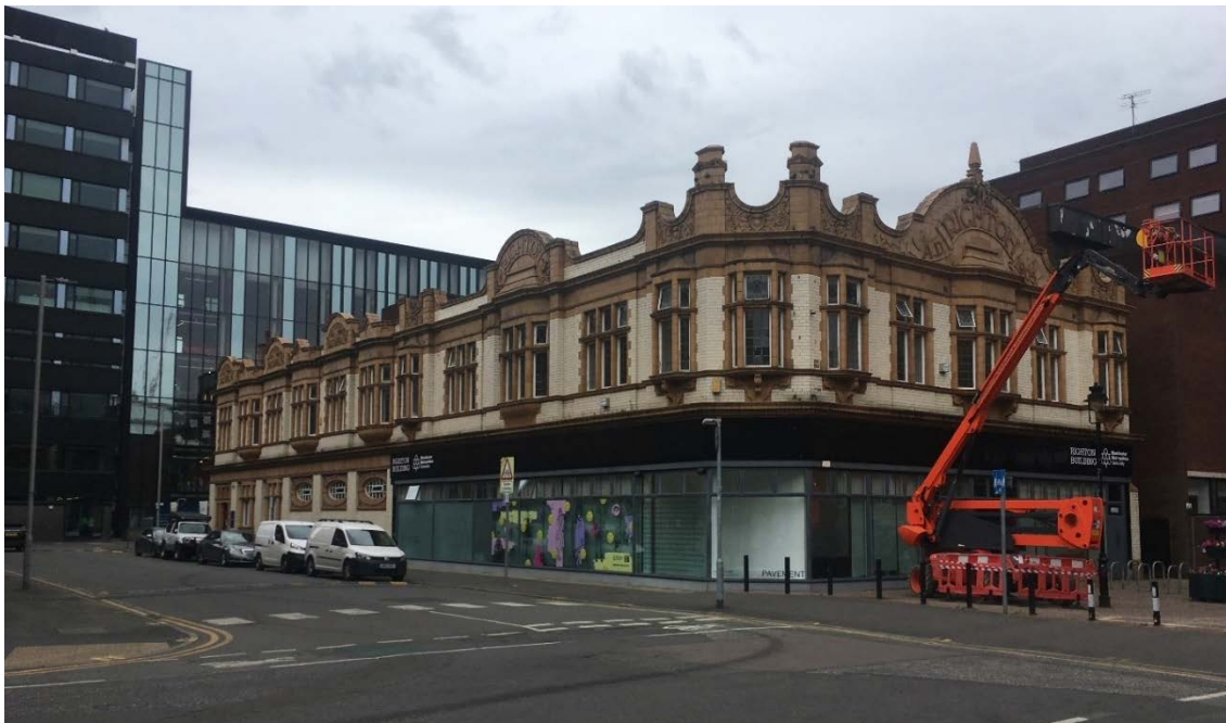
Figure 1: The Righton Building as viewed from Cavendish Street (Source: SLHA 2022).
