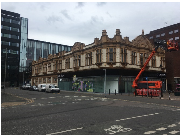
Figure 32: General view of the building from the north east showing the primary north and east elevations with the buff terracotta and glazed brick, note the non-original shopfronts and signage.
