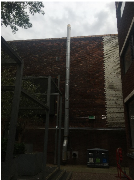
Figure 36: View of the existing external flue to the west elevation .
