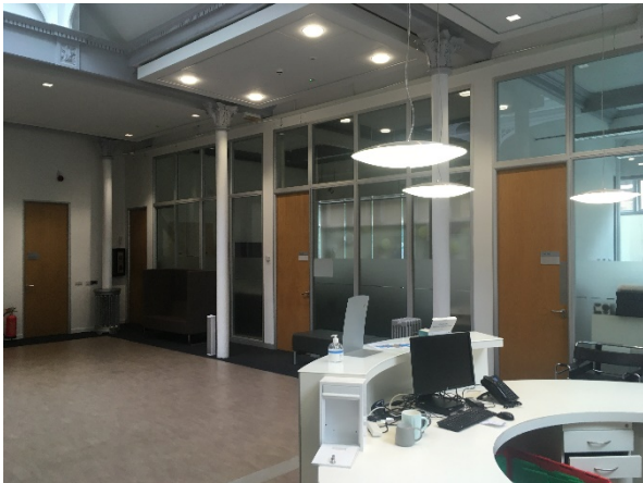
Figure 30: View again of the modern glazed partitions to the eastern side of the floorplan. Also note the modern floor and ceiling finishes.
