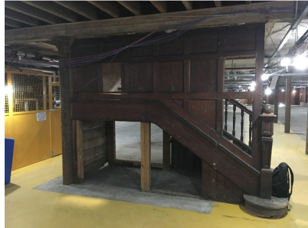
Figure 21: Timber stair that connects the primary ground floor area to the basement. Although this was down to the storage / backroom space the timber staircase is equally as ornate as the timber stair between ground and first floor.
