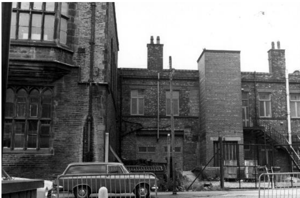
Figure 19: The rear (south) of the building seen in 1973 shortly before the demolition of the Cavendish Street Sunday school (left) was demolished. Note the introduction of a modern brick goods lift. Also note the introduction of the (white) flue pipe that has now been removed but which cut through the decorative cill and cornice. (Source: Manchester Archives)
