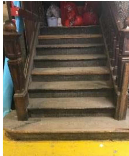
Figure 23: The primary timber stair survives albeit in poor condition.
