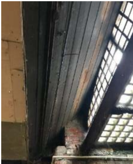
Figure 22: View of a pavement light with internal timber boarding. The arrangement was to maximise natural daylight within the basement.
