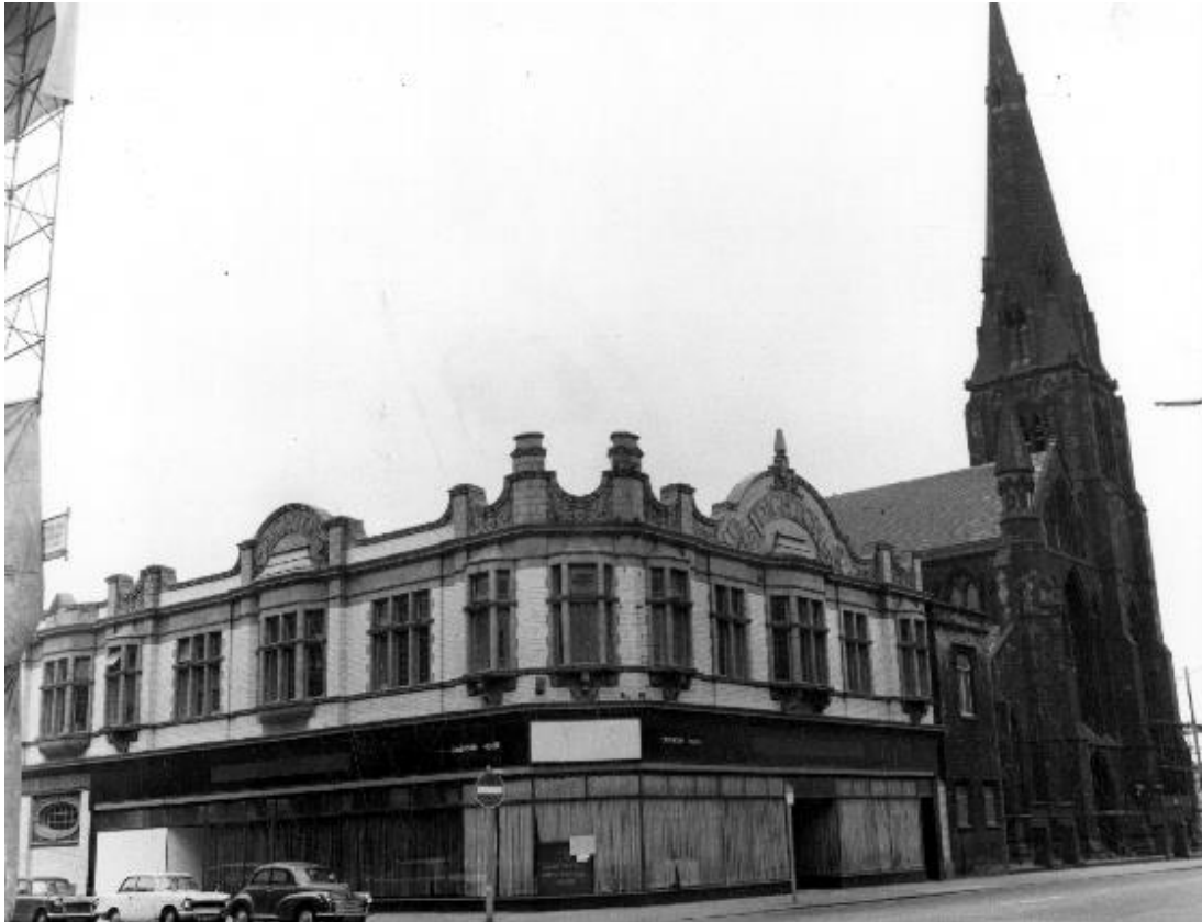
Figure 18: The Righton Building as seen in 1973 shortly before the Cavendish Street Chapel was demolished. (Source: Manchester Archives)
