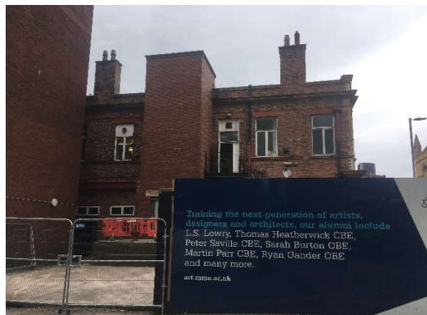
Figure 33: The compromised south elevation with external service lift.
