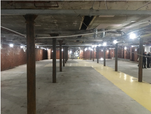
Figure 20: View of the basement following clearance of the modern storage furniture in March 2022.
