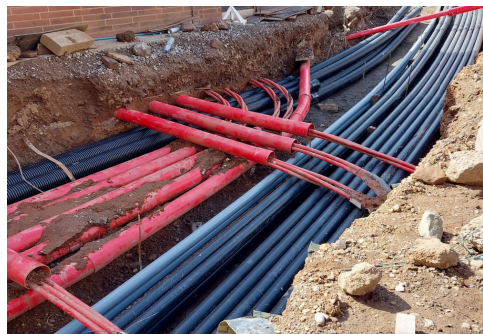
Site photographs - installation of underground services
