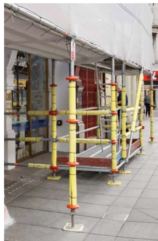
Proposed Pavement Lift Protection Method
