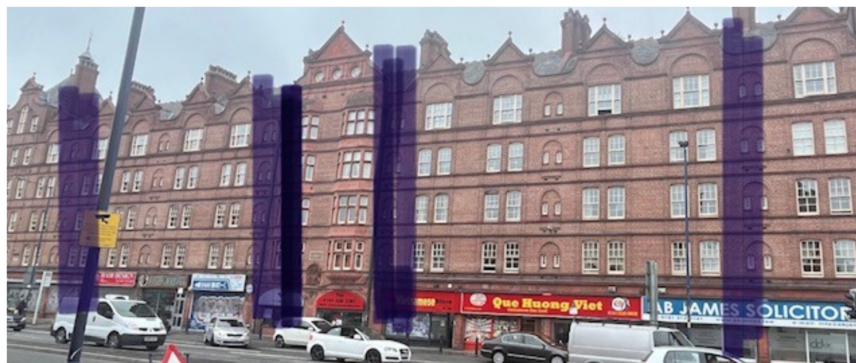
Planned Location of Tower Scaffolds
