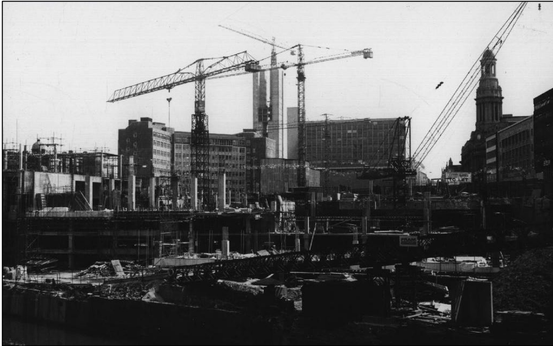
Plate 17: Development on site of Deansgate Hotel, the Arndale centre can be seen in background 1973
