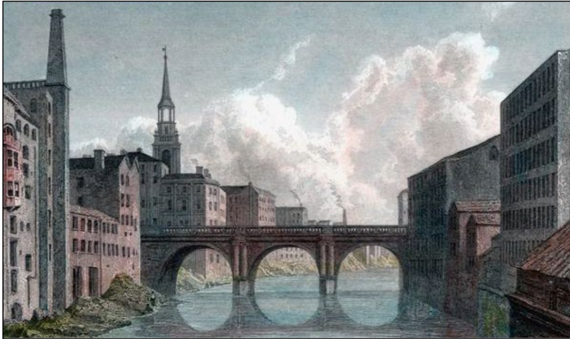
Plate 5: Blackfriars Bridge, Manchester, by Westall, 1829
