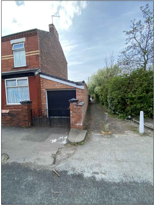
FRONT VIEW TOWARDS No.24
