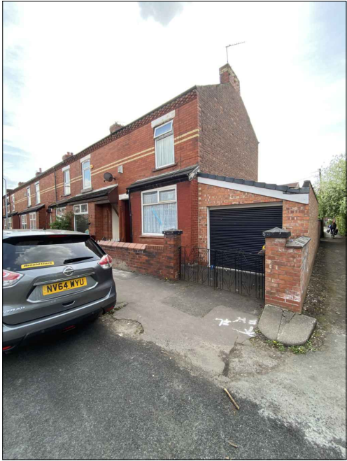
FRONT VIEW TOWARDS No.24
