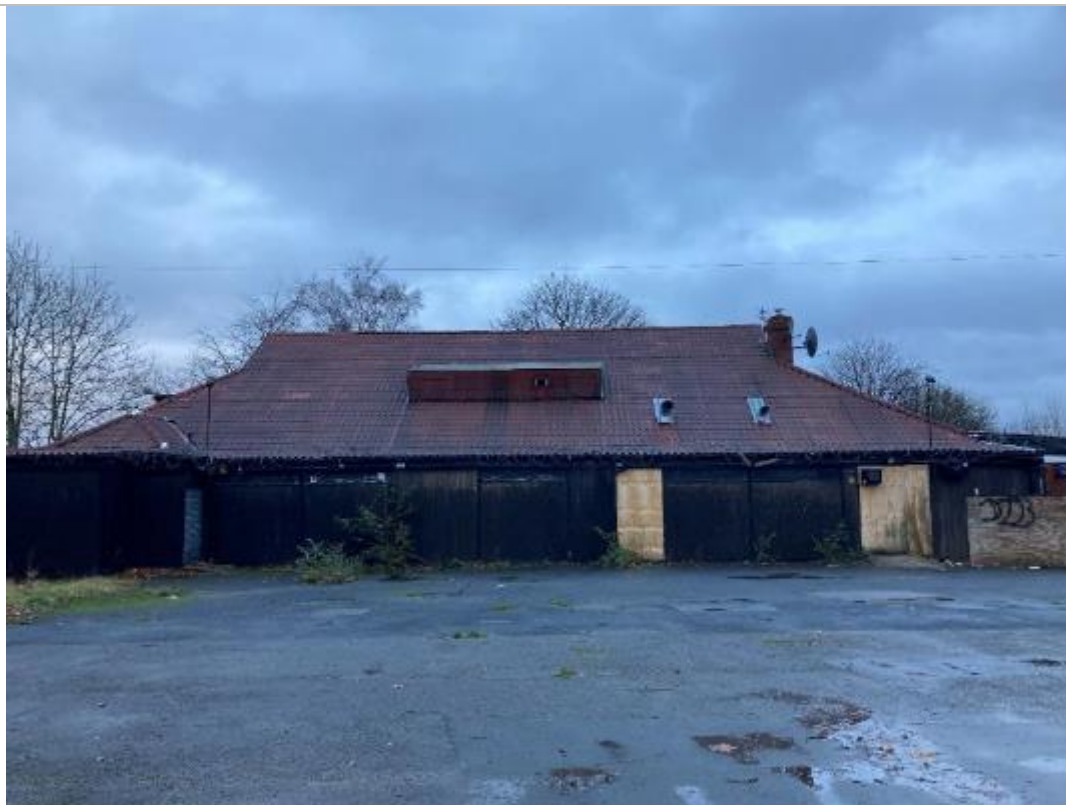
PLATE 3 VIEW OF SITE FACING NORTH
