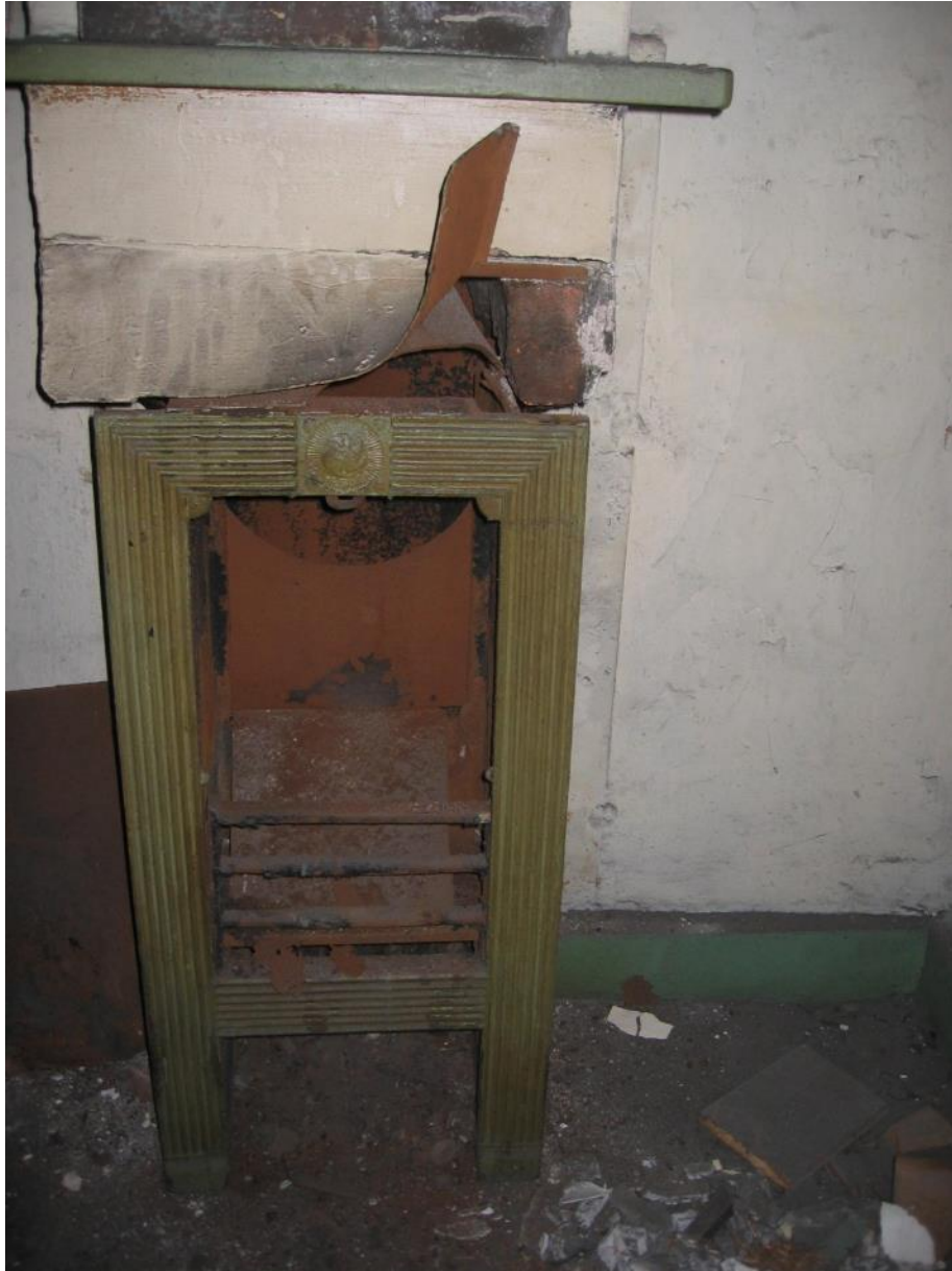
Figure 89: Room A05 (looking west) – This image shows an unusual design of an 18 th century cast iron projecting fireplace found on the western elevation (Source: SLHA 2007).
