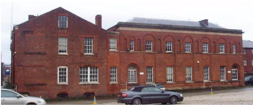
Figure 98: The west elevation as seen in 2007, showing the 18 th century dwelling to the left, the 1842-43 office extension to the right, and later, narrow link in-between. (Source: SLHA 2007)
