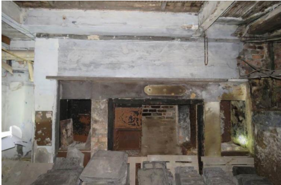
Figure 73: Room B07 (looking west) – This room was originally the main kitchen for the eastern dwelling, and has not been used since the late-19 th century. This very lofty room retains the original 18 th century stone surrounds to the former kitchen range, along with parts of the original/early cast iron range/ovens and mechanical spit. (Source: SLHA 2017)
