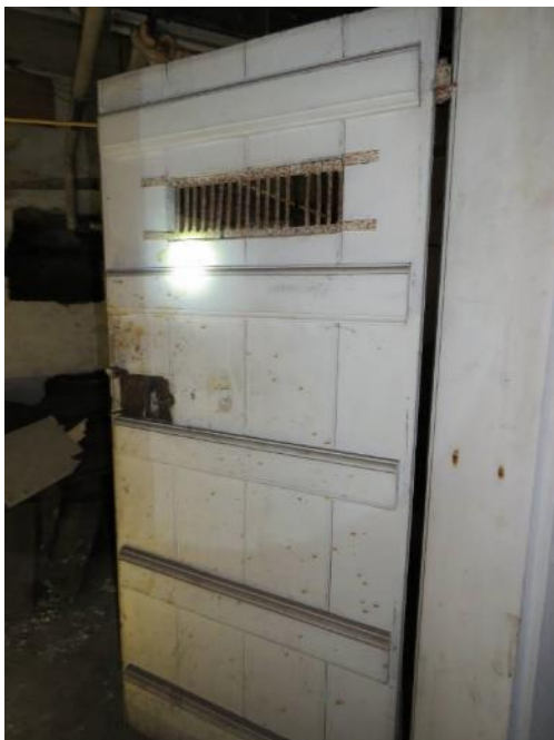
Figure 74: Room B06 - The 18 th century battened door into the original wine cellar of the eastern dwelling, including original iron grill. Above this door are the remains of the original 18 th century servants bell board (Room B01). (Source: SLHA 2017)
