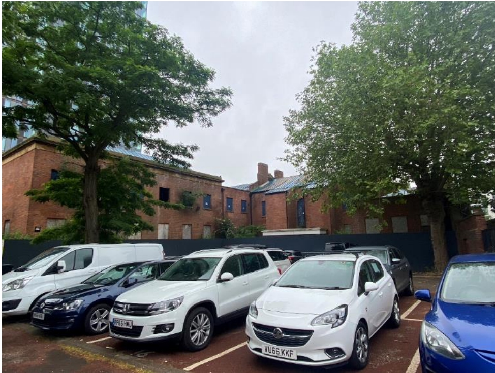
Figure 104a: The current appearance of the rear elevation of the building (Source: Watch This Space (Jembrana) Ltd 2022)
