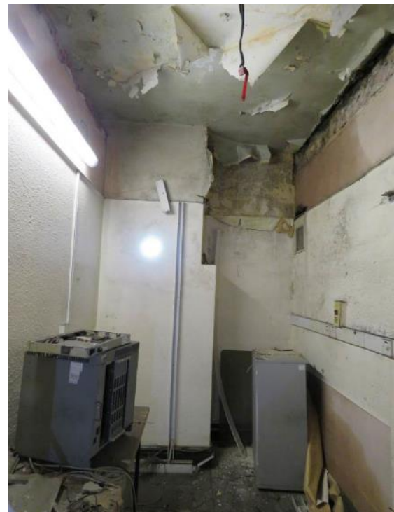
Figure 72: Room F31 (looking east) – This room forms part of one of the rear bedrooms of the western dwelling before the link corridor was inserted. (Source: SLHA 2017)
