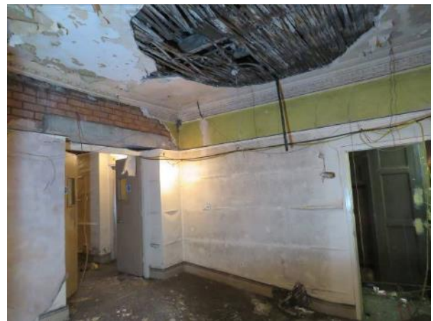
Figure 69: Room F16 (looking south-west) showing the entrance into the original servant's attic stairs (right) (Source: SLHA 2017)
