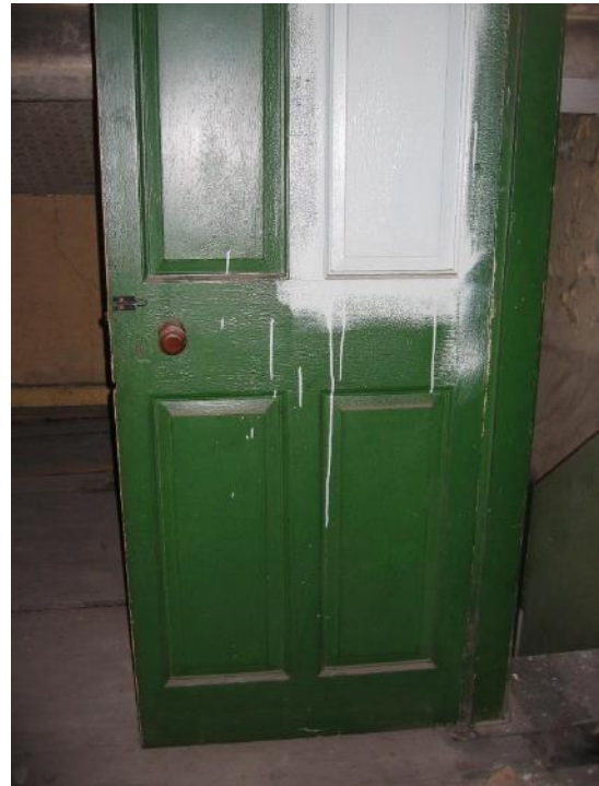
Figure 97: The original panelled door into Room A02 (Source: SLHA 2007)
