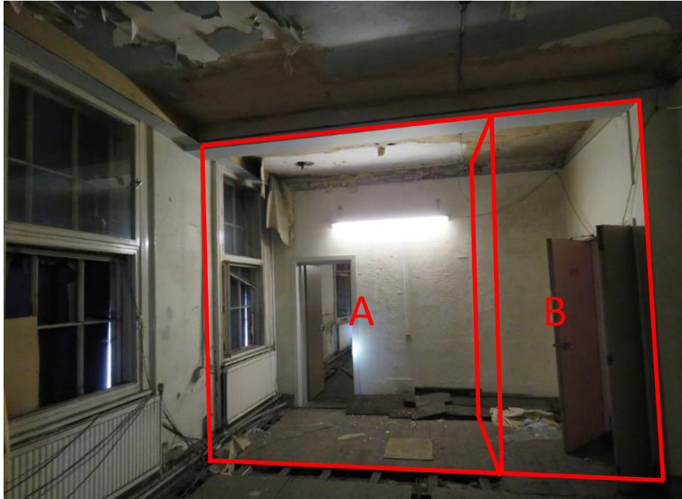
Figure 65: Looking towards the eastern end of Room F17– This room was originally two rooms (as mirrored in the eastern dwelling and below in the former entrance halls). The small room to the left (A) was likely originally a dressing room accessed from one or both principal front bedrooms.
