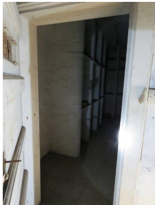
Figure 75: Looking into the original 18 th century wine cellar (Room B06), complete with brick wine shelves. (Source: SLHA 2017)
