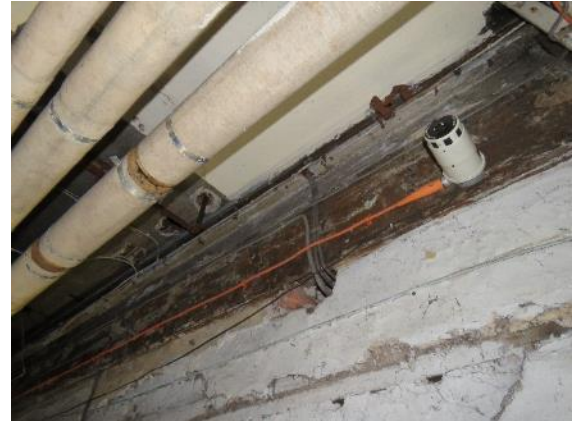
Figure 75b: The remains of the original 18 th century servant's bell board (Source: SLHA 2017)
