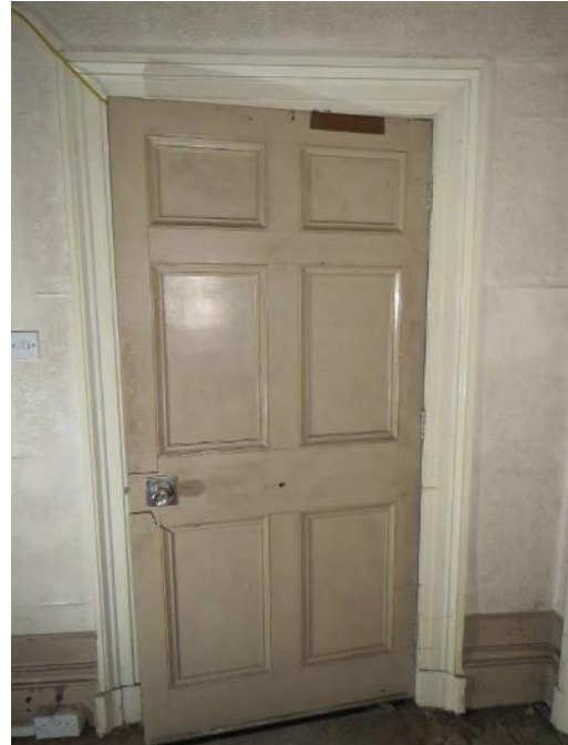
Figure 55: Detail of the original door from entrance hall to staircase hall (Room G02) (Source: SLHA 2017 – please note the condition of the building has significantly worsened since 2007)
