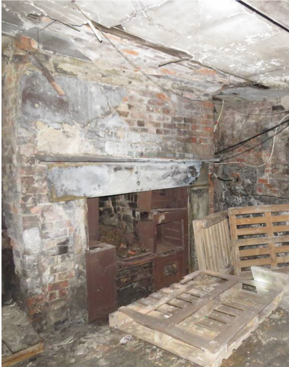
Figure 79: Room B12 (looking south) - This room would probably have formed the scullery to the main kitchen of the western dwelling, and retains a surviving 19 th century cast iron kitchen range and stone surround. (Source: SLHA 2017)
