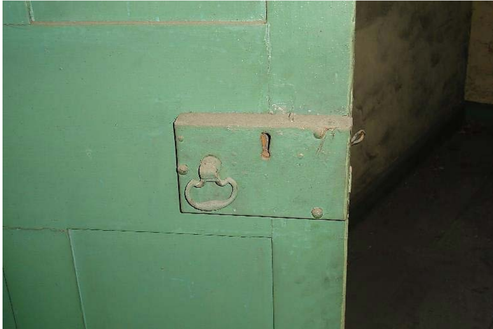
Figure 90: Room A05 (looking north) – This image shows an example of an original 18 th century panelled door and rim lock with surviving brass Dutch drop handle. (Source: SLHA 2007)
