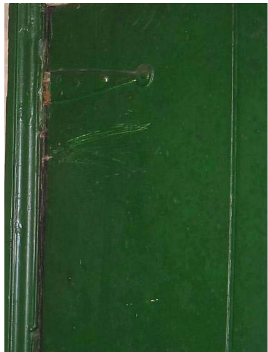
Figure 95: Detail of the two 18 th century hand-forged, iron butterfly hinges to the attic access hatch (Source: SLHA 2007)
