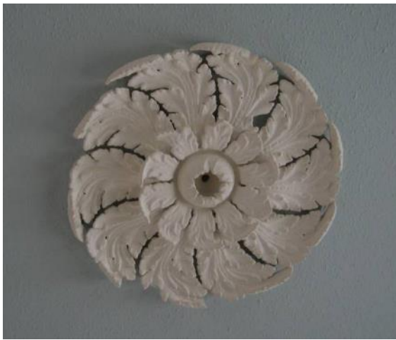
Figure 56: The heavily detailed original/early plaster ceiling rose as it appeared in Room G04 in 2007. (Source: SLHA 2007)
