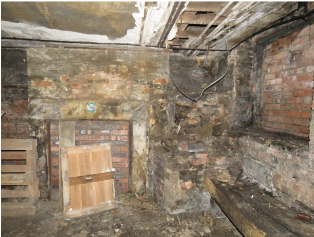
Figure 76: Room B11 (looking west) -This room would have formed the washhouse connected to the main kitchen of the western dwelling, and retains its 18 th century stone fire surround, stone sink and brick and stone corner 'copper' (fire heated clothes washing tub). (Source: SLHA 2017)
