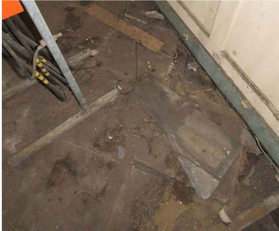
Figure 62: The original stone flag floor in Room G02. (Source: SLHA 2017)
