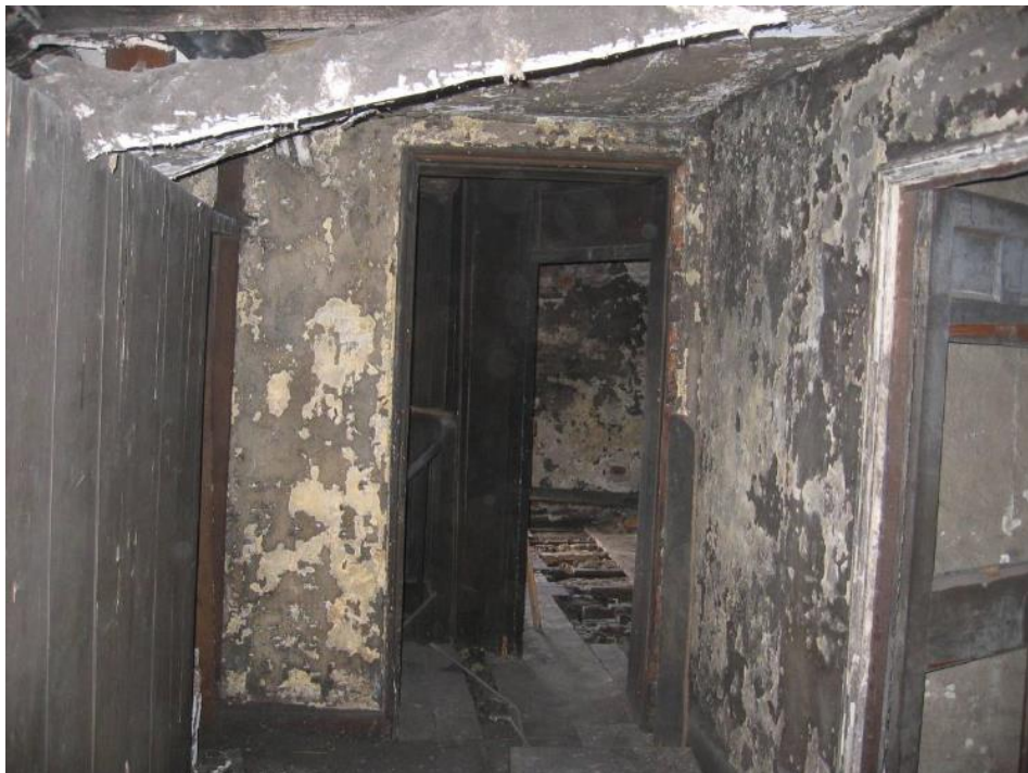
Figure 82: Room A15 (looking west) – This room forms the attic landing and corridor of the western dwelling and would have originally been used as servant's accommodation. This attic space, and the three rooms leading off have not been decorated since the 19 th century, and retain early paint schemes, original doors/architrave and skirting. (Source: SLHA 2007 - please note the condition of the building has significantly worsened since 2007)
