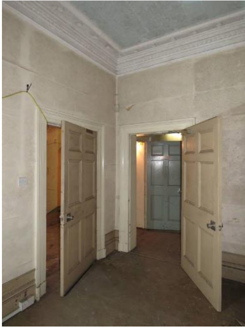
Figure 54: The south-west corner of Room G04, showing the two original 18 th century doors/architraves forming the original door from entrance hall to staircase hall (left – Room G02) and door from entrance hall into second reception room (right-G05). (Source: SLHA 2017 – please note the condition of the building has significantly worsened since 2007)
