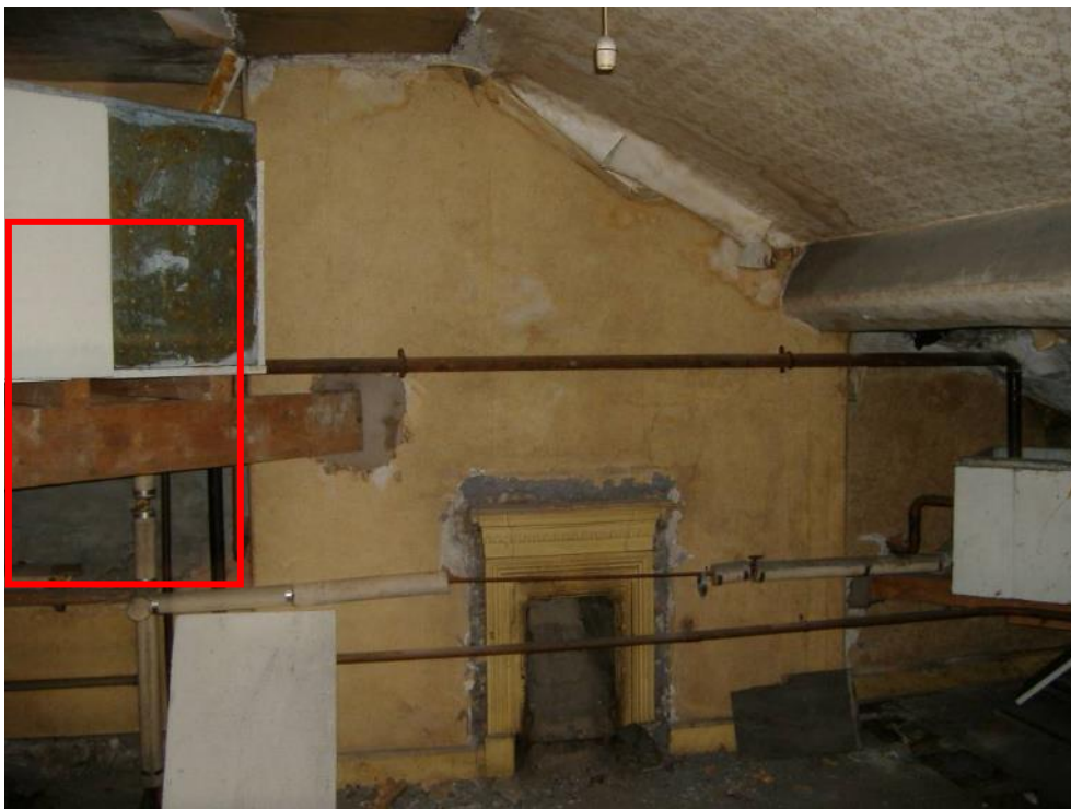
Figure 91: Room A02 (looking east) showing a 19 th century cast iron fire surround and 19 th century “sanitary” ceiling wallpaper. Note the now blocked window outlined (left), as seen in Figure 22 & 42. (Source: SLHA 2017 - please note the condition of the building has significantly worsened since 2017)
