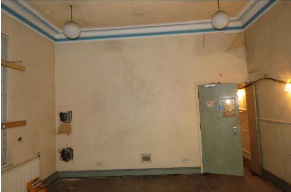
Figure 58: Room G03 (looking west) – This simpler room formed one of two original rear rooms, and was substantially altered to create a link corridor between the two former dwellings (right) in the late-19th century and is likely to have received the current plaster cornice in this period. The original open fireplace was blocked (note air vent cover) and the narrow alcove to the left covered in 1977 (Source: SLHA 2007 – please note the condition of the building has significantly worsened since 2007)
