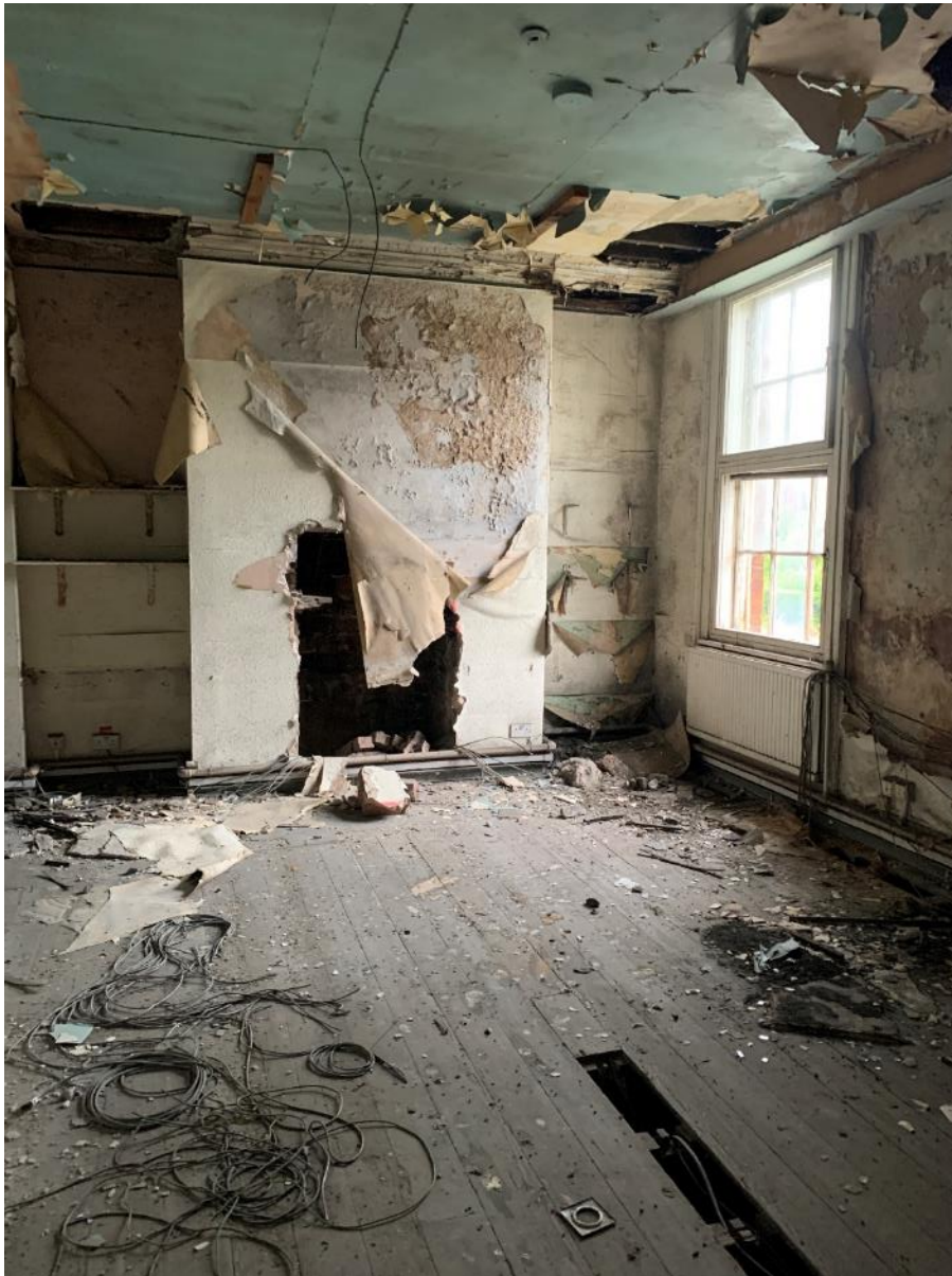
Figure 64: Room F17 (looking west) – This room retains areas of plain 18 th century plaster cornice (Source: Watch This Space (Jembrana) Ltd 2022)
