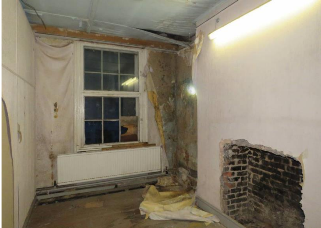
Figure 70: Room F22 (looking north) – this room was originally part of the adjacent Room F21, but subdivided in the 20 th century. (Source: SLHA 2017 - please note the condition of the building has significantly worsened since 2007)
