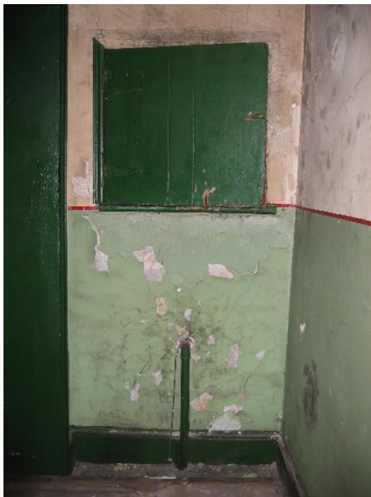
Figure 94: Original 18 th century battened access hatch into the roof void from A03. This door retains two 18 th century hand-forged, iron butterfly hinges. (Source: SLHA 2007 - please note the condition of the building has significantly worsened since 2007)
