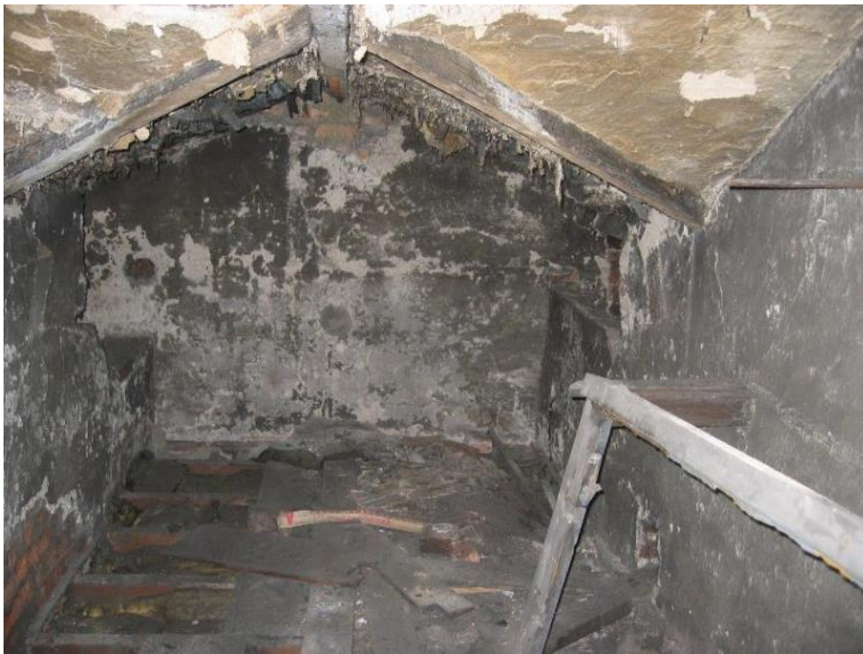
Figure 84: Room A14 (looking north) - Looking into the windowless central attic room, which is located within the central pediment of the western dwelling. Originally there was a small glazed rooflight which has since been covered. The two small openings to the left and right lead into the roof voids. (Source: SLHA 2007 - please note the condition of the building has significantly worsened since 2007)
