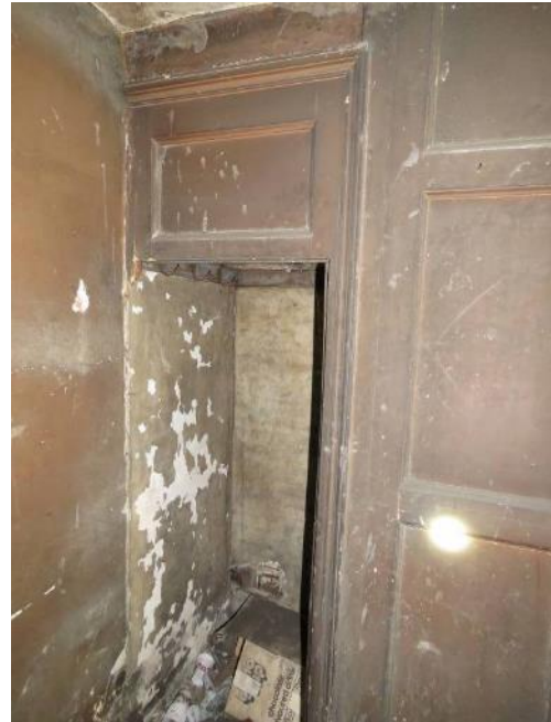
Figure 80 & 81: Room F34 (looking west) – The remaining 18 th century timber panelling and staircase from the original landing area of the western dwelling (Room F16) into the attic and servant's accommodation above. (Source: SLHA 2017)
