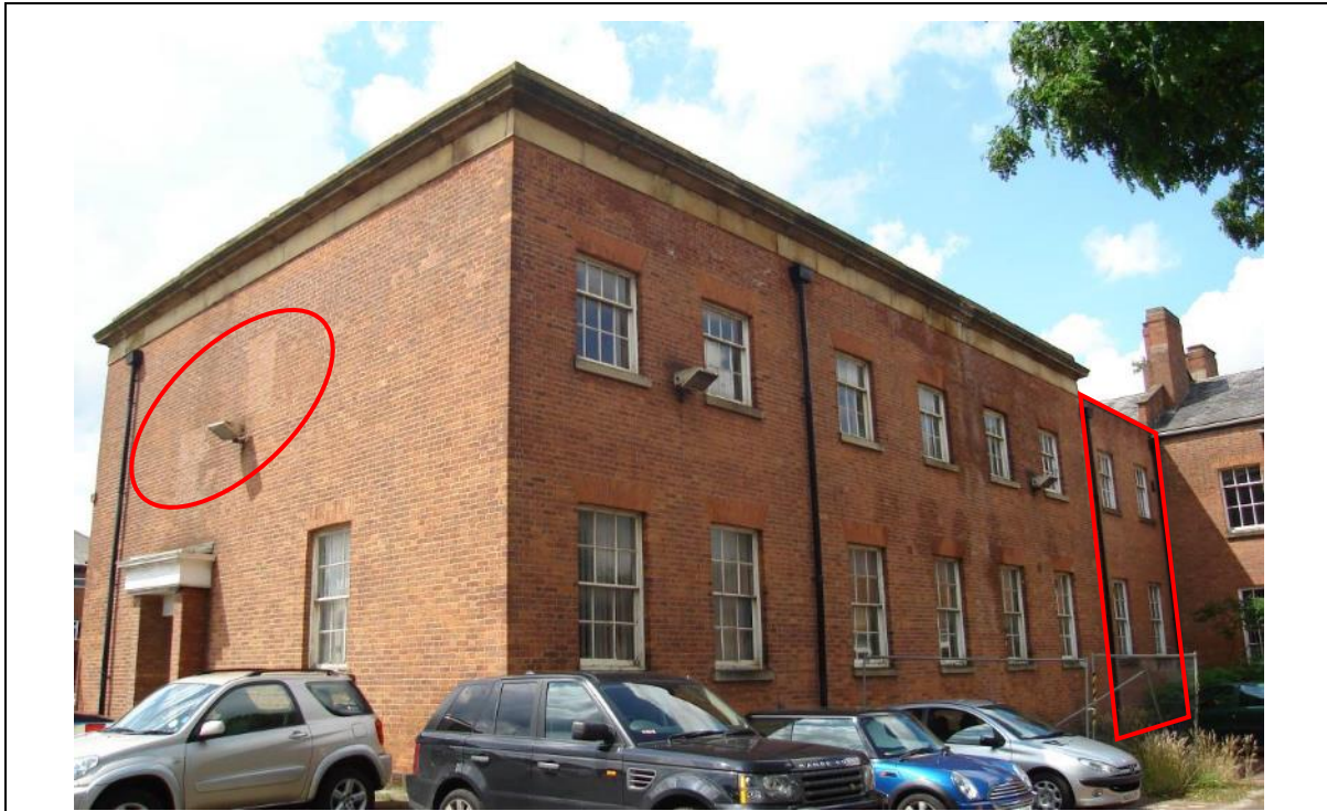
Figure 102: The east (right) and south (left) elevations of the 1842-3 office extension as seen in 2007, showing the 1977 alterations, including the infilling of the two original small windows (left) and addition of two-storey matching link in the location of the original office staircase and toilets (outlined right).
