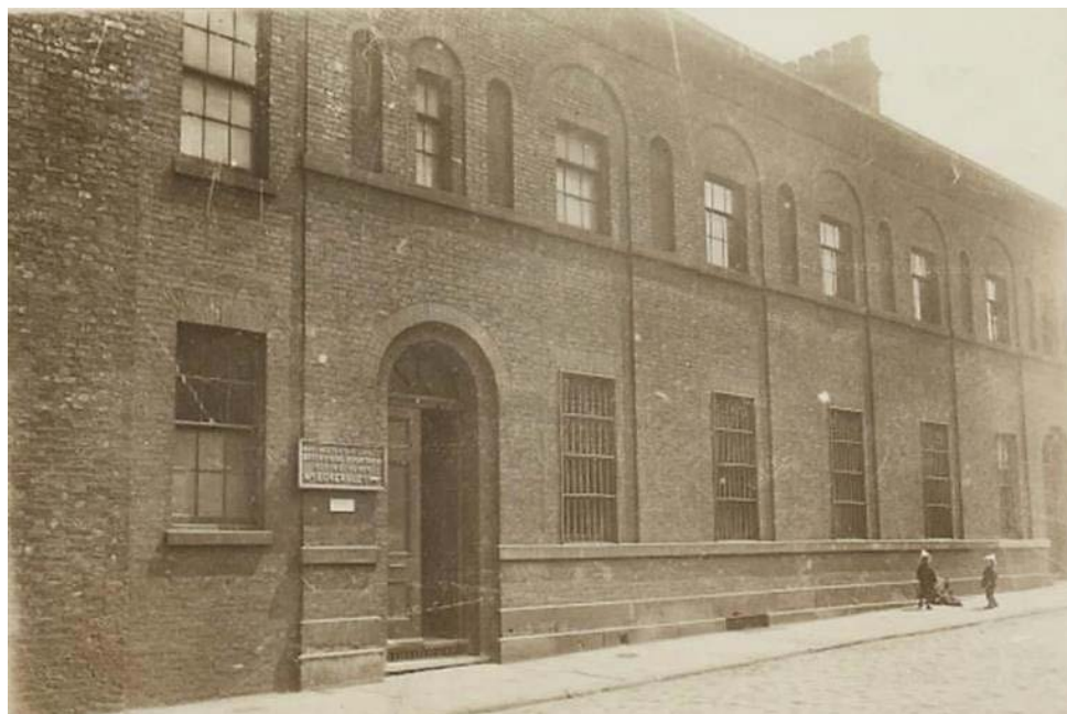
Figure 99: The principal west elevation of the 1842-3 Bridgewater Trustees Office, as seen when used by the Manchester Ship Canal in c1920 (Source: Canal & Rivers Trust)
