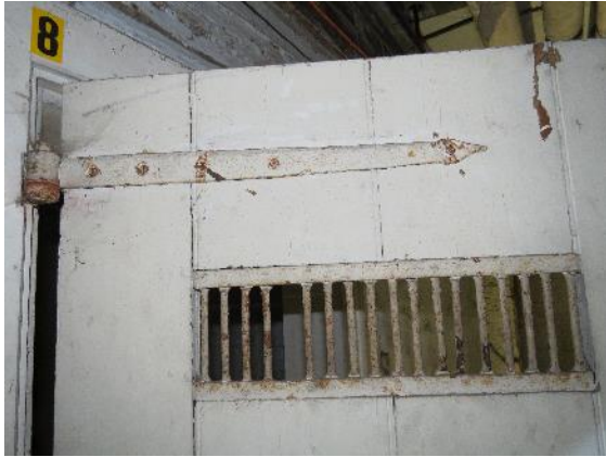
Figure 75a: Detail of the 18 th century handmade iron hinges to the wine cellar door. (Source: SLHA 2017)
