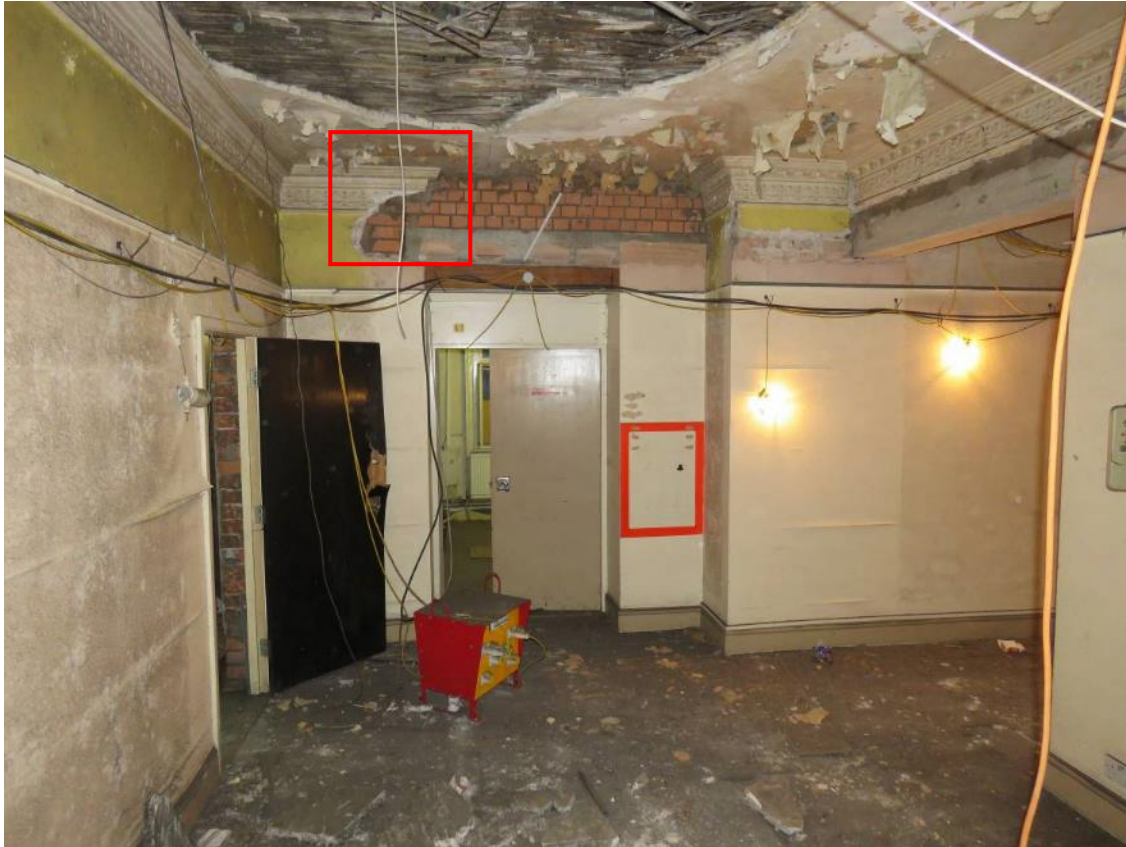
Figure 67: Room F16 (looking north) – This room was originally the landing of the western dwelling. The north wall shows evidence of the 1977 infilling of the original extension/alcove which gave access into the former dressing room (marked B in Figure 66 above). Note the return section of original plaster cornice denoting the corner of this now blocked alcove (outlined). (Source: SLHA 2017 - please note the condition of the building has significantly worsened since 2007)
