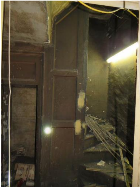
Figure 80 & 81: Room F34 (looking west) – The remaining 18 th century timber panelling and staircase from the original landing area of the western dwelling (Room F16) into the attic and servant's accommodation above. (Source: SLHA 2017)
