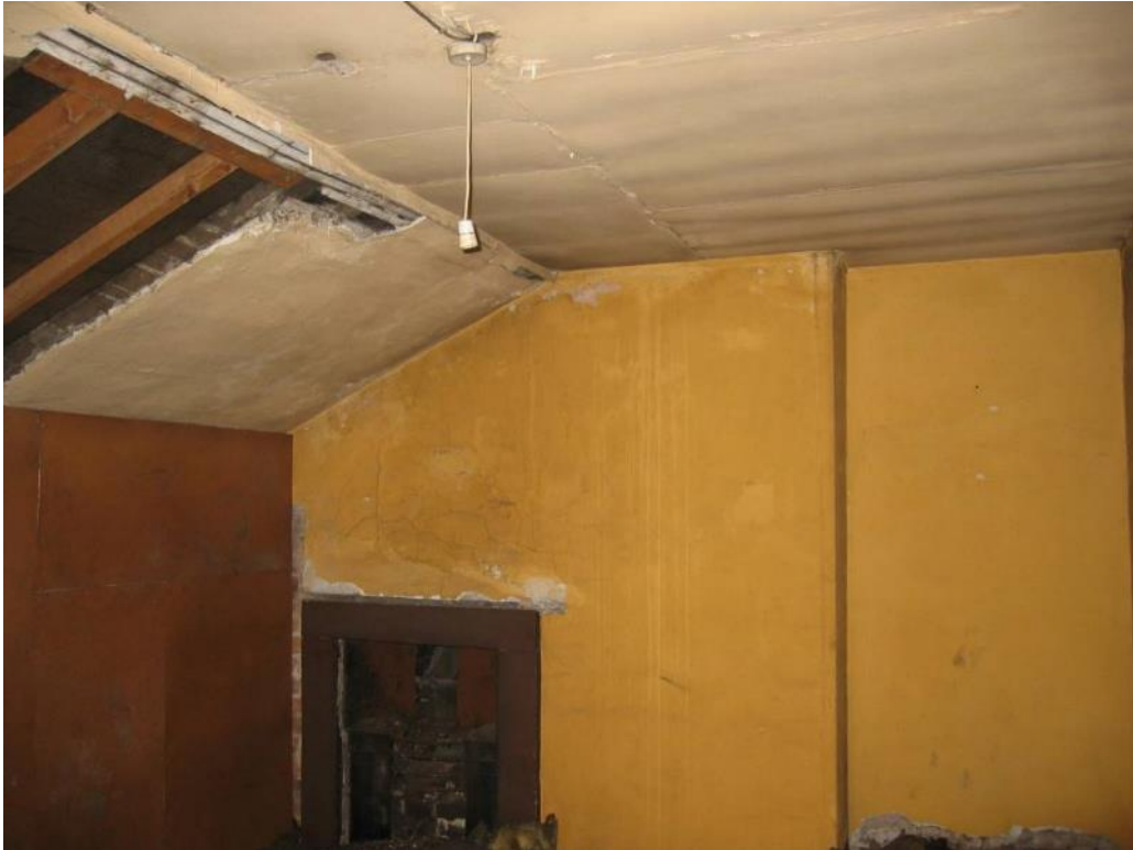
Figure 87: Room A06 (looking west) – This image shows a surviving original 18th century cast iron register grate and fire surround. (Source: SLHA 2017 - please note the condition of the building has significantly worsened since 2017)
