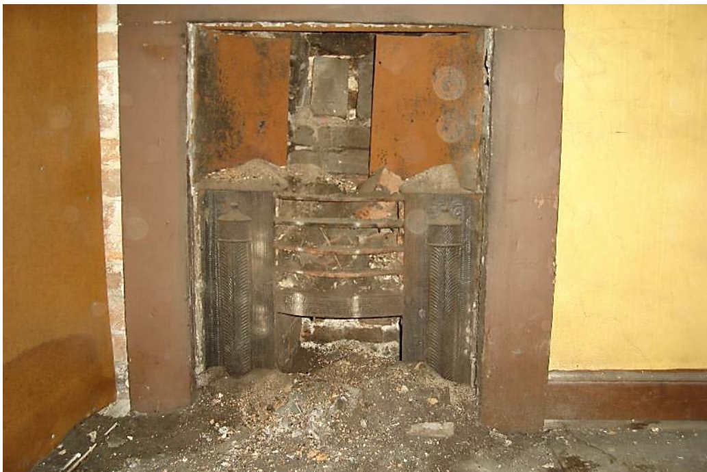
Figure 88: Room A06 (looking west) – Detail of the surviving original 18th century cast iron register grate and fire surround. (Source: SLHA 2017)
