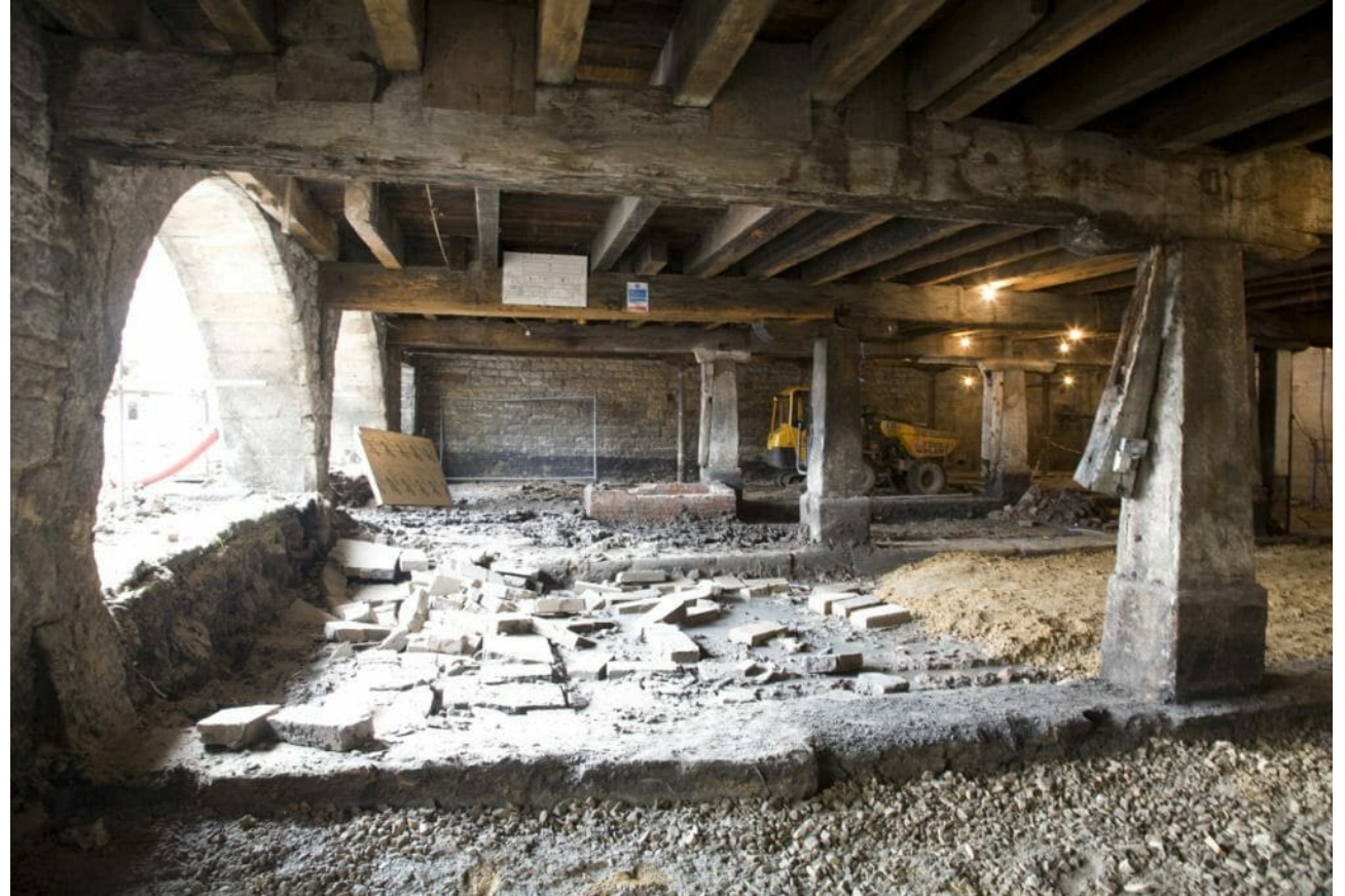
2.2.17 Basement boat bays, prior to conversion, undated (Northern Quarter Manchester)
