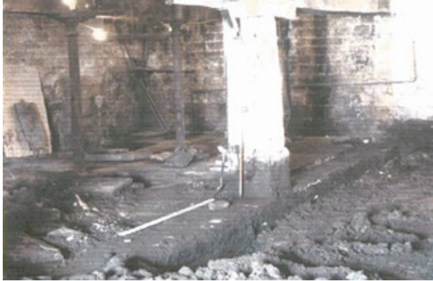
2.2.16 Basement prior to conversion, 2006 (University of Manchester)
