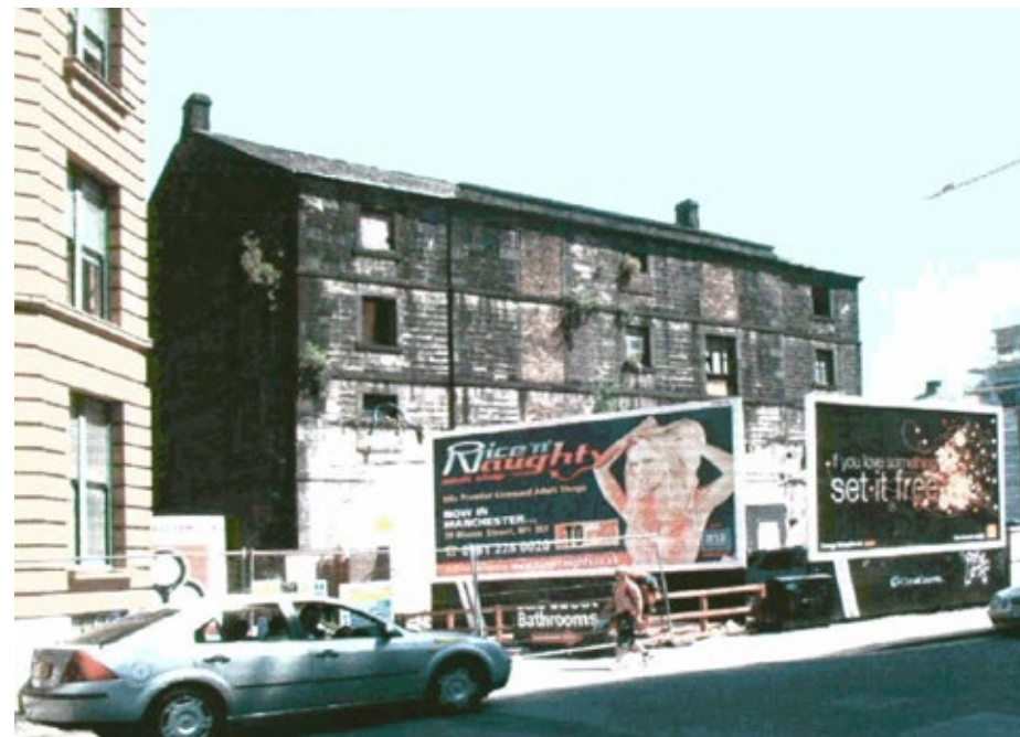
2.2.12 West elevation with loading doors, partly obscured by hoardings, 2006 (University of Manchester)
