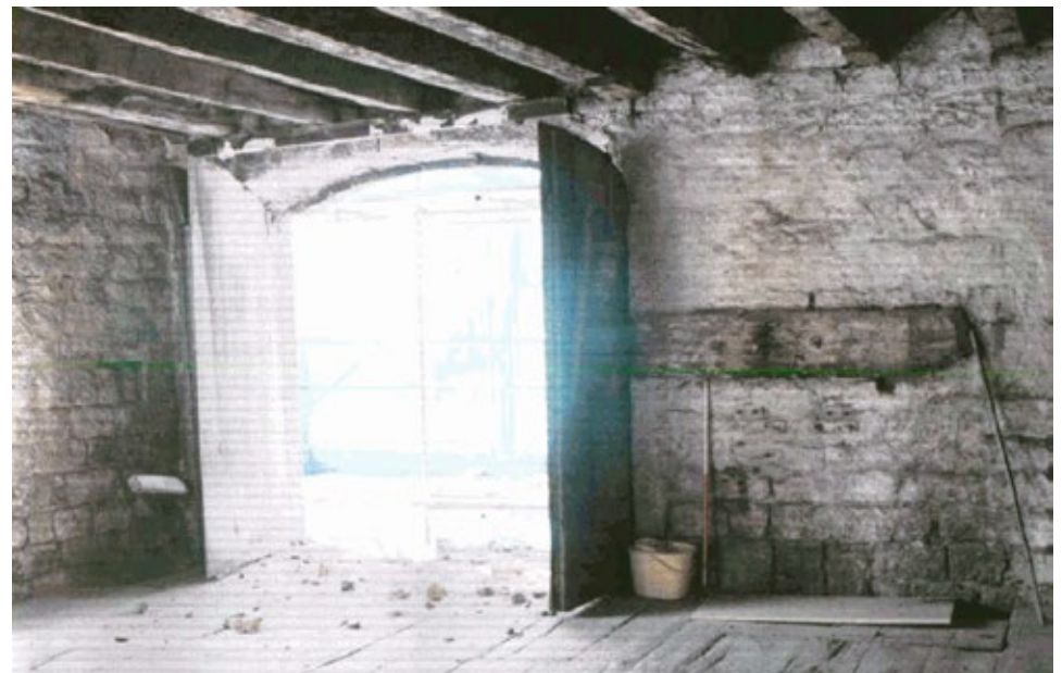
2.2.23 Ground floor loading door to the west elevation, 2006 (University of Manchester)
