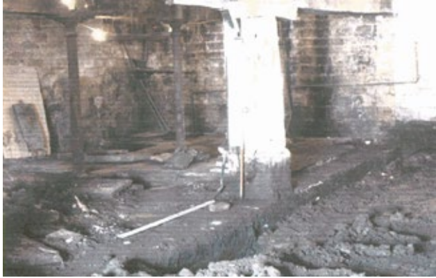
2.2.19 Basement pillars and columns, 2006 (University of Manchester)
