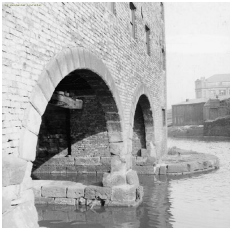
2.1.9 Boat bays to Dale (Carver's) Warehouse, date unknown but prior to infill (Manchester Libraries)
