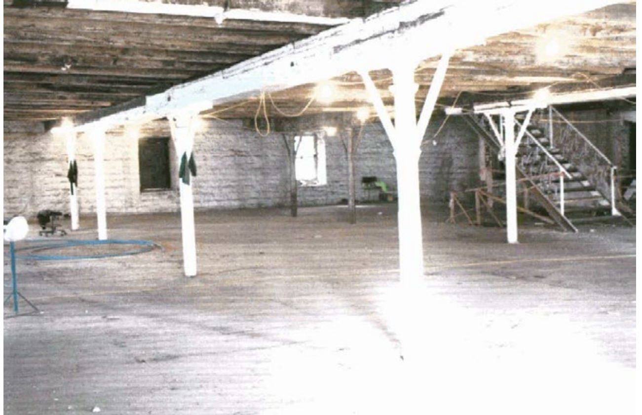
2.2.21 Ground floor, showing the principal stairs and the cast-iron columns with beams above, 2006 (University of Manchester)
