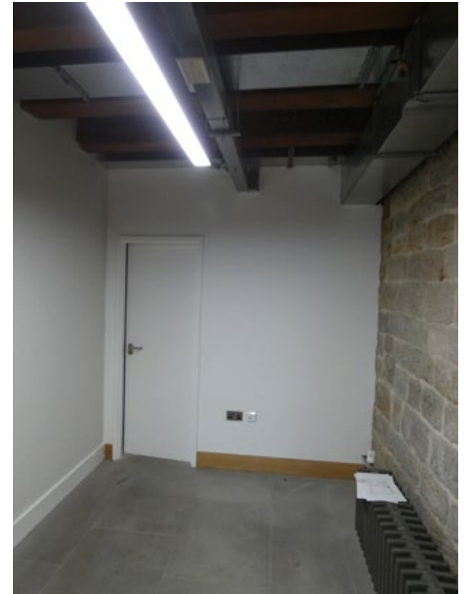
3.3.1.1 View of store room in NW corner (Insalls)
