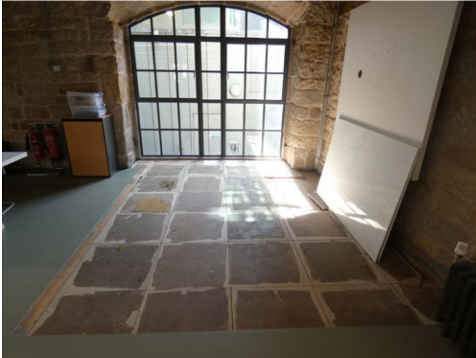
3.3.2.6 View of office interior NW corner, Ground Floor (Insall)
