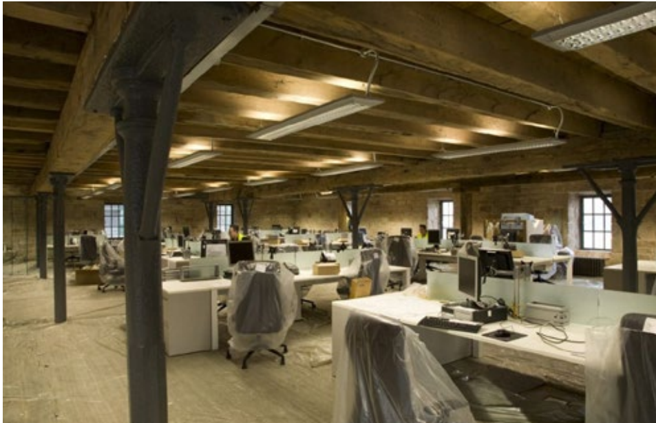
2.2.28 Restoration complete, with retention of cast-iron columns, undated (c.2008) (Northern Quarter Manchester)
