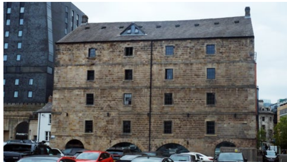
3.2.4 View of east elevation from the former canal basin (Insalls)
