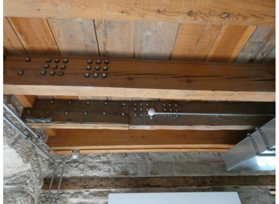
3.3.2.7 View of ceiling structure in the NW corner, Ground Floor (Insall)
