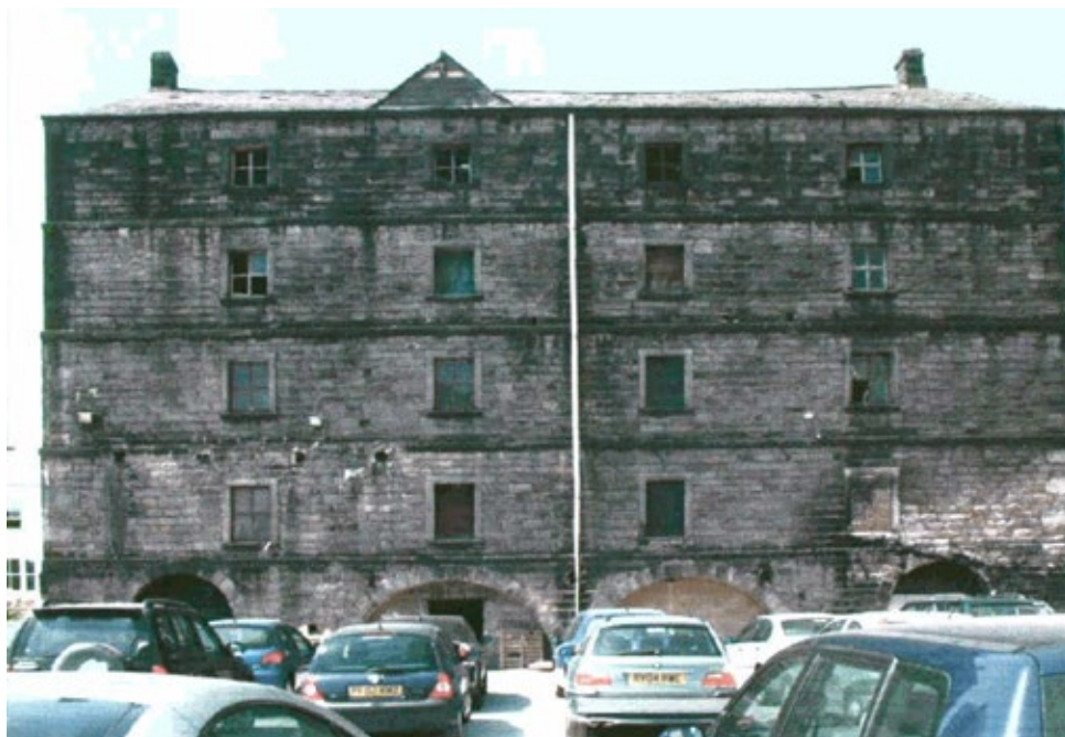
2.2.11 East elevation with boat bay openings infilled, 2006 (University of Manchester)
