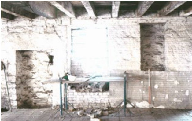
2.2.20 Integral cupboards surviving in the west wall at ground floor, 2006 (University of Manchester)
