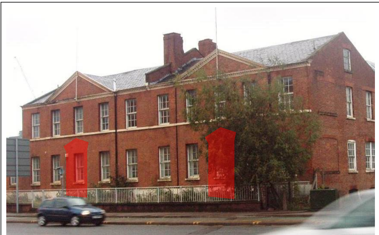
Figure 35: The north elevation as seen in 2007, showing the location of the original front entrances into both dwellings shaded red. (Source: SLHA 2007 – Note the current condition of the building has since worsened)
