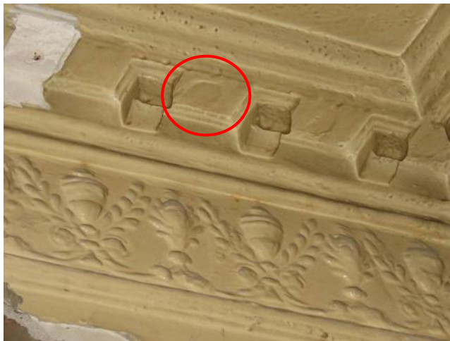
Figure 49 & 50: The original cornice surviving in Room G12 showing missing rosettes (left), and surviving cornice with rosettes within the adjacent Room G11 (right) (Source: SLHA 2017)
