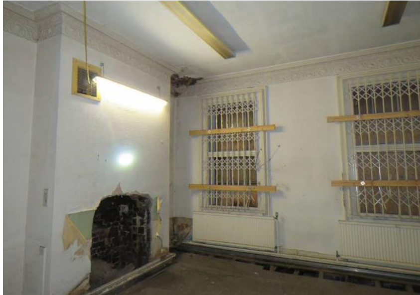
Figure 46: Room G11 (looking north) – Formally one of two reception rooms within the western dwelling, the room retains all its 18 th century plaster cornice of urns and wreaths. (Source: SLHA 2017)
