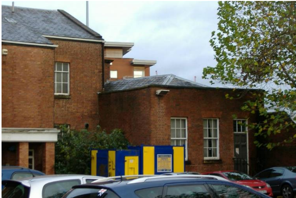
Figure 41: The southern aspect of the mid-to-late 19 th century single-storey extension, which formed the "Porch Office". The door to the single storey wing was inserted in 1977, whilst the two window openings were inserted in 1985. (Source: SLHA 2007 – Note the current condition of the building has since worsened)
