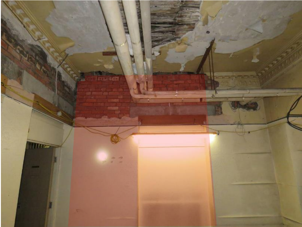
Figure 48: Room G12 (looking north) – This room was the original 18 th century hallway for the western dwelling, which opened out into the entrance hall shown in Figure 47 above. To the south was originally a now demolished separate staircase hall. The room retains parts of its 18 th century cornice, which features urns, laurel leaves and brackets with indentations from former, now removed plaster rosettes, surviving examples of these can still be seen in Room G11 (see Figures 49-50) (Source: SLHA 2017)
