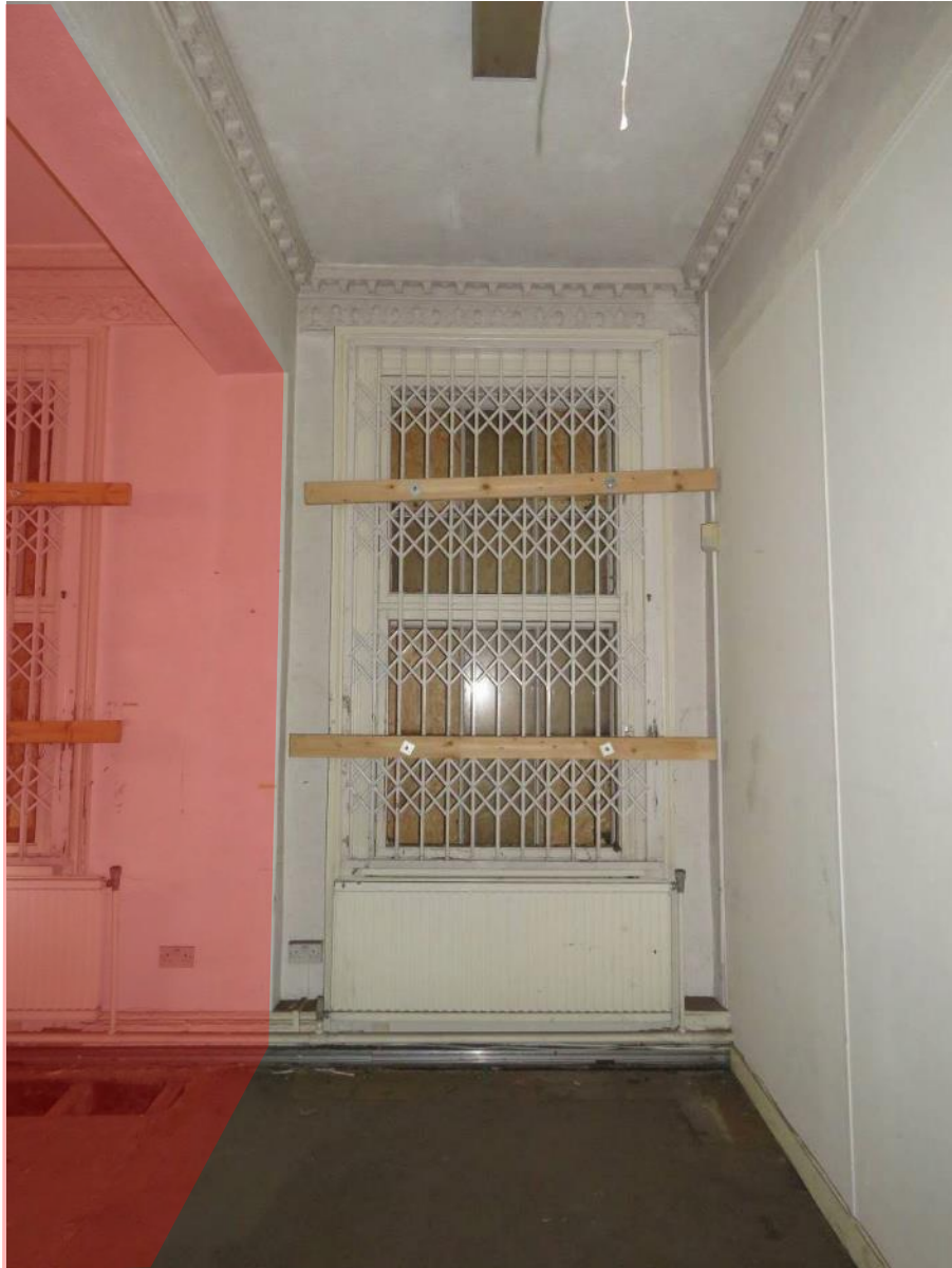
Figure 47: Room G11 (looking north) – This room was the original entrance hall and was originally divided from the room pictured above by a dividing wall (indicated by red shading). The window was inserted following the removal of the front entrance door in the late-19 th century.
