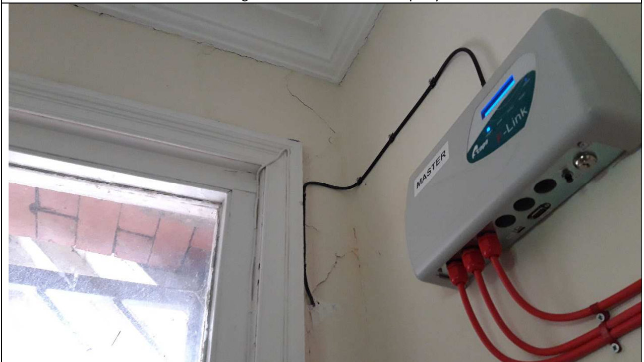
Minor Cracking in Lobby Over Front Access Door
