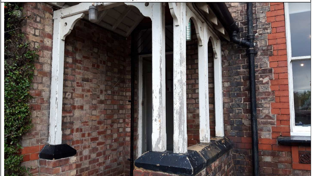
Paint Breakdown to Front Porch
