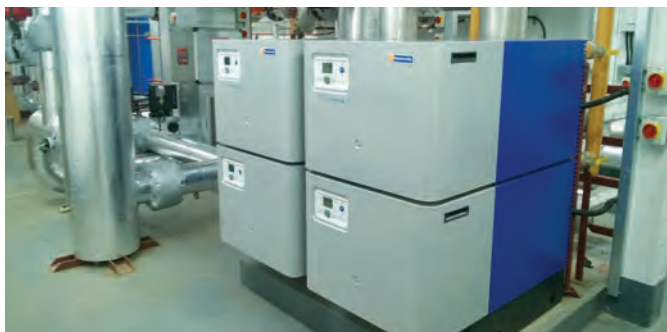
Two Wessex ModuMax mk3 WM254/508V boilers now heat the whole cathedral up within one day, compared to a week by the previous boilers.
