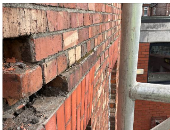
Opening up works to investigate movement in rear wall.
