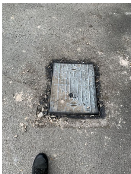
Photograph 8: Evidence of below ground services and drains identified.
