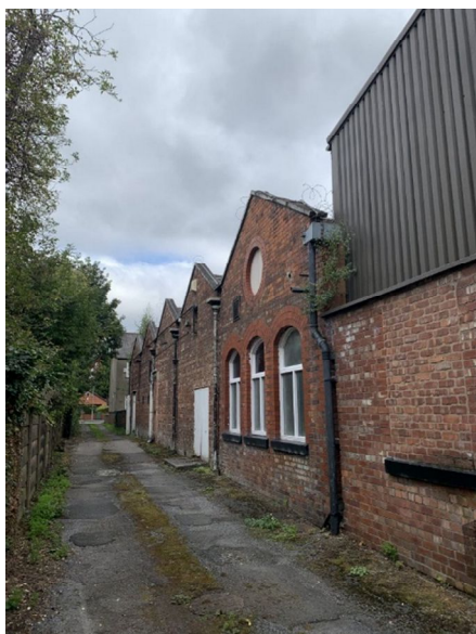
Photograph 1: View of site access road and the north façade of the existing building.
