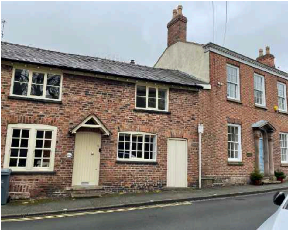
2 View looking north-east towards the Georgian south wing of Northen House
