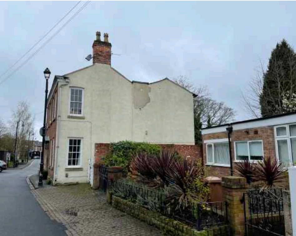
4 View looking west along Ford Lane towards Northern House
