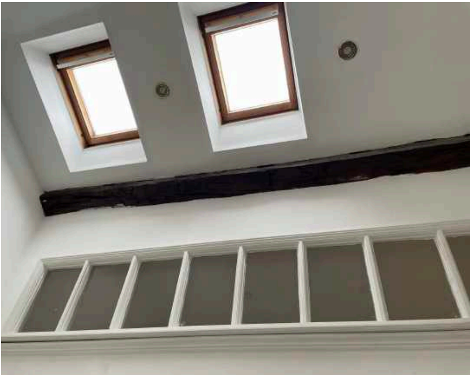
1 View looking towards the roof lights and high level window providing light into the En-suite
