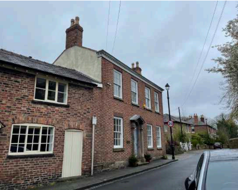
1 View looking north-east towards the Georgian south wing of Northen House
