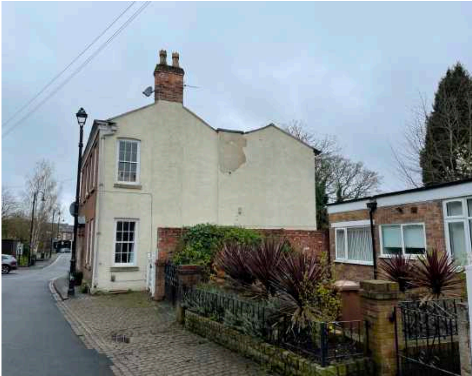
3 View looking west along Ford Lane towards Northen House
