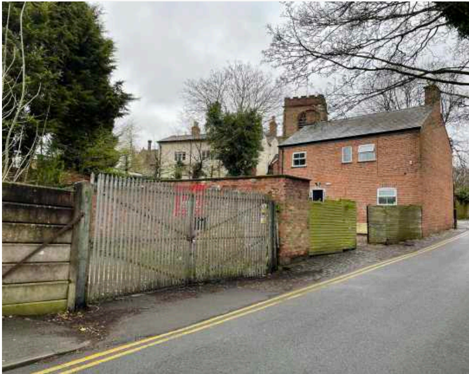
5 View looking west from Boat Lane towards Northern House from outside the Scrap Yard site
