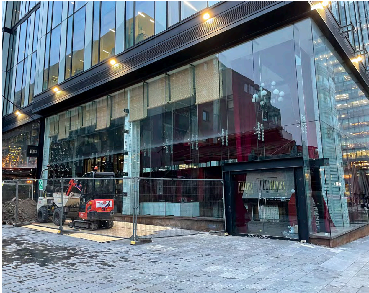
The existing building following removal of the existing external terrace
