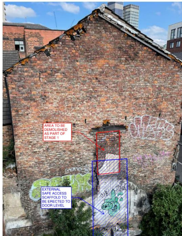
Image: Stage 1 Demolition Area
