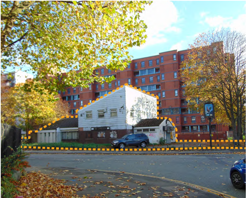
Existing Building on site
