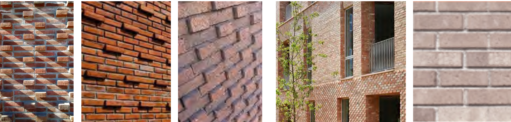
Projecting Brick Bond Texture
