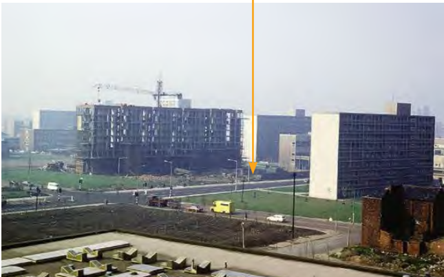
Cooper House under construction 1973
