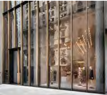
Capped Curtain Wall
