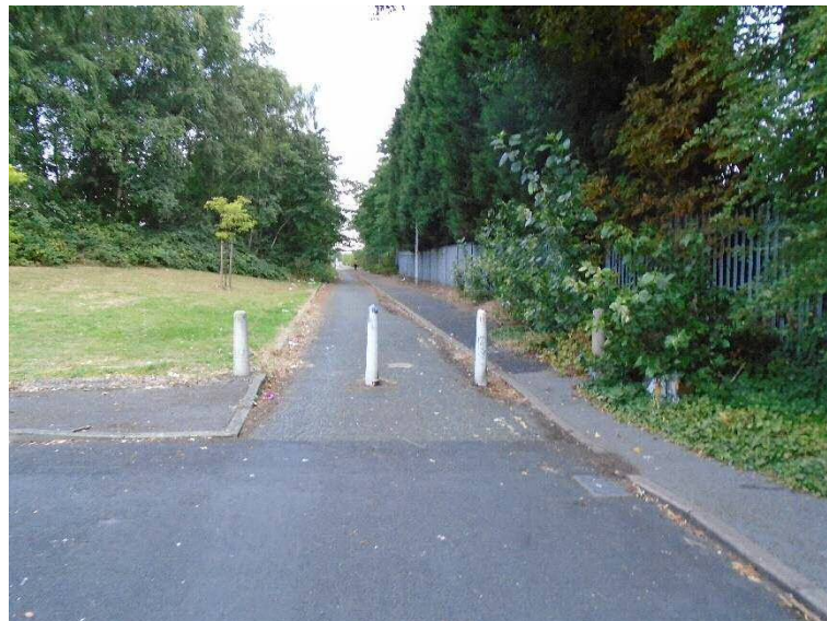
Photo 6: Redgate Lane Cycle Path
