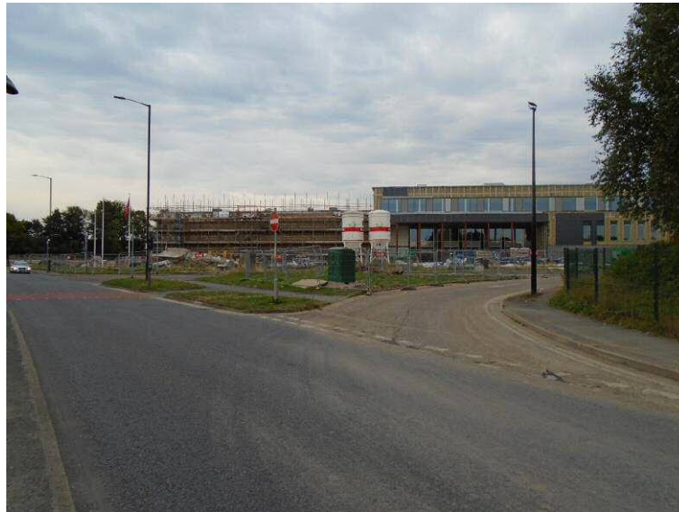
Photo 1: Hyde Road Access Junction (Prior to the Approved Amendments)
