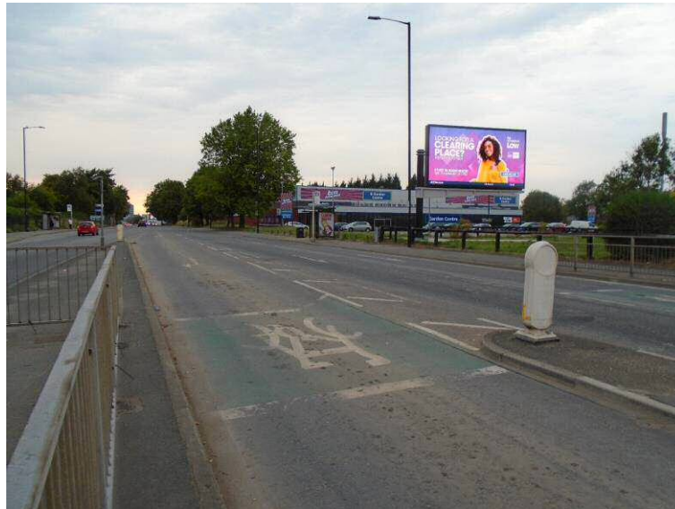
Photo 7: Advanced Stop Line (ASL) at the Hyde Road/Belle Vue Street Junction
