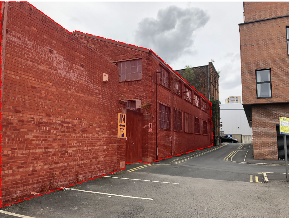
IMAGE 004- BROCK STREET - Extent of demolition from Brock Street
