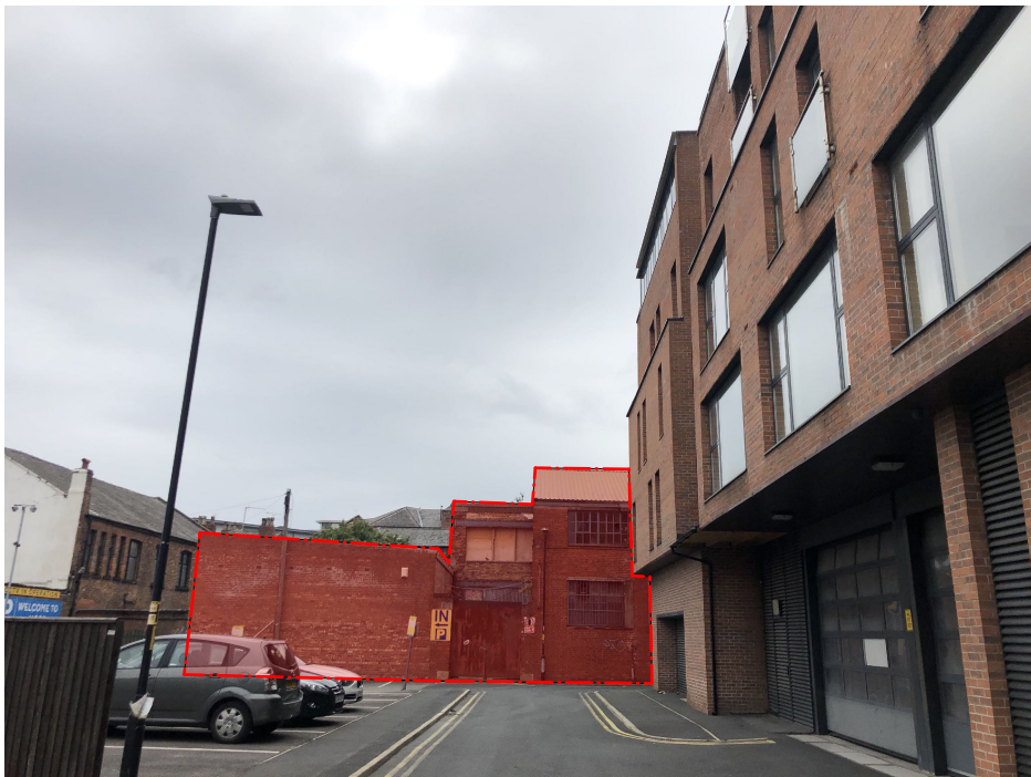
IMAGE 003- BROCK STREET - Extent of demolition from Lomax Street
