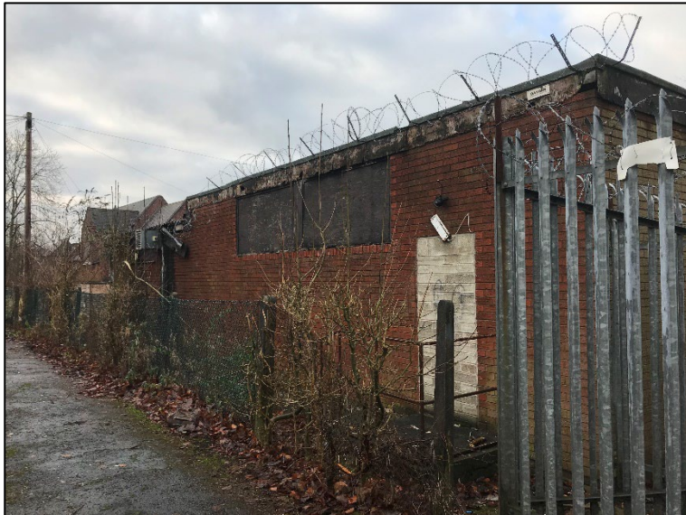
Photograph 4.2 South-east face of building 1
