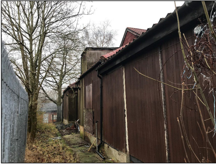
Photograph 4.4 North-west face of building 1
