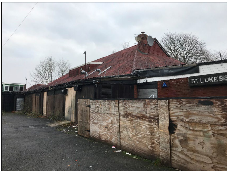
Photograph 4.3 South-west face of building 1
