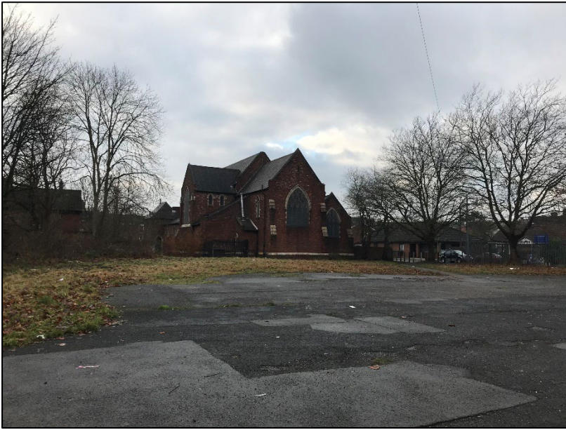
Photograph 3.1 Overview of site, view south-west
