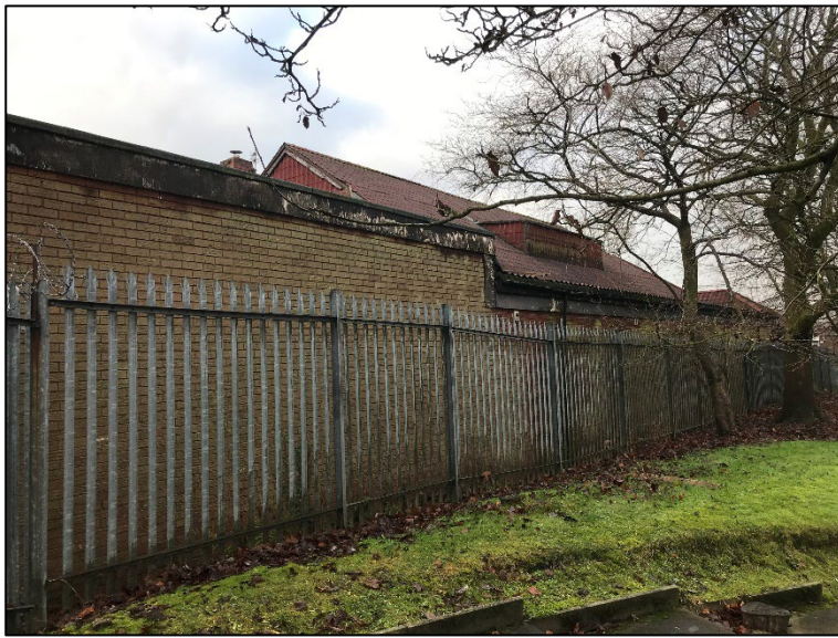
Photograph 4.1 North-east face of building 1
