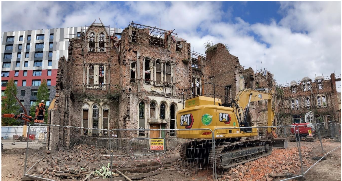
Condition of Existing Walls during demolition and enabling works
