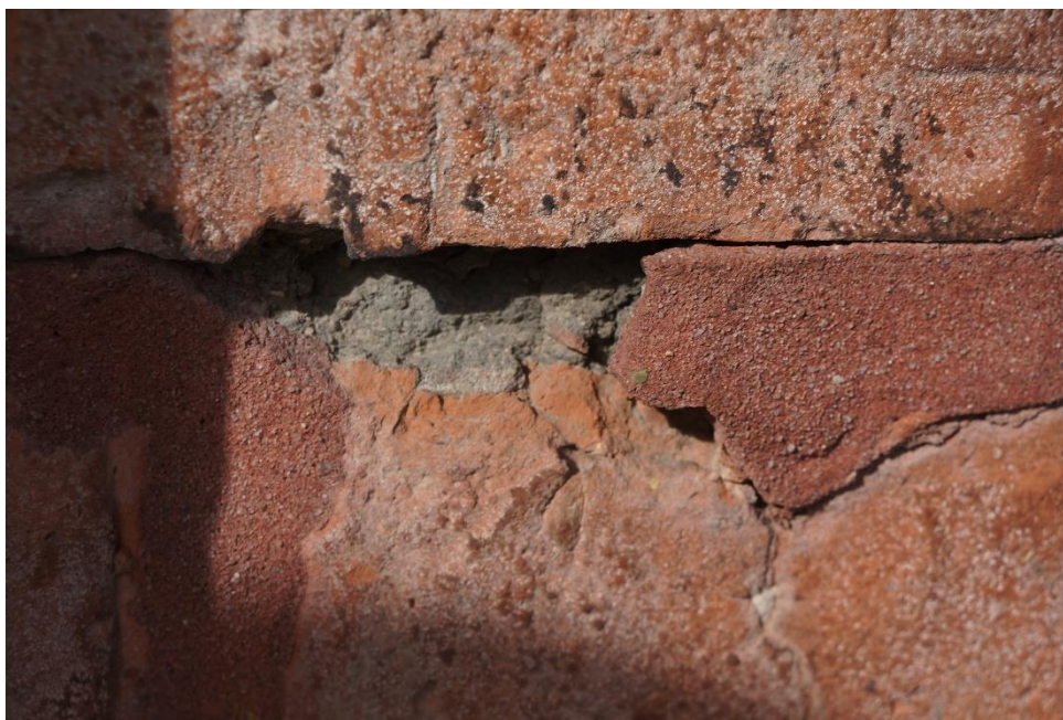
Evidence of original and later mortar samples
