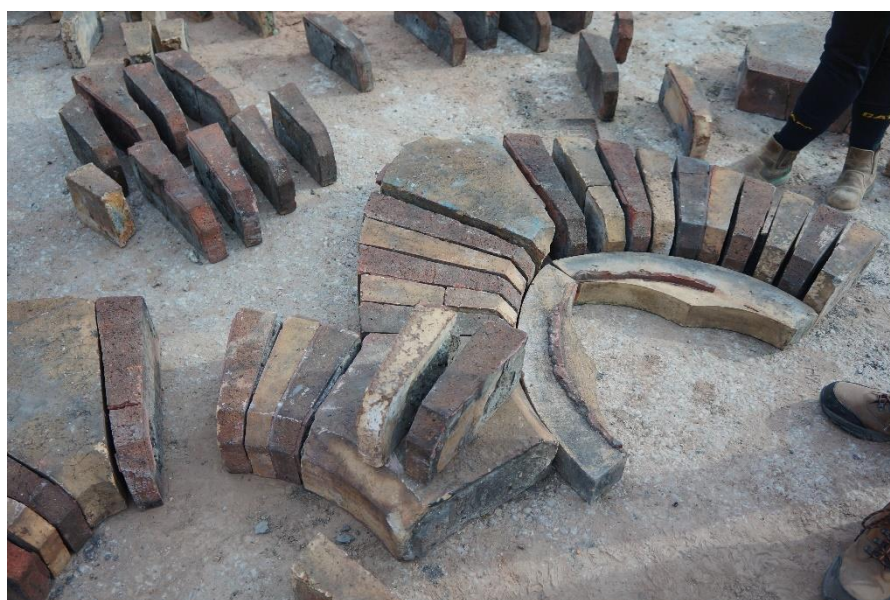
Evidence of abrasive cleaning to polychromatic Voussoirs
