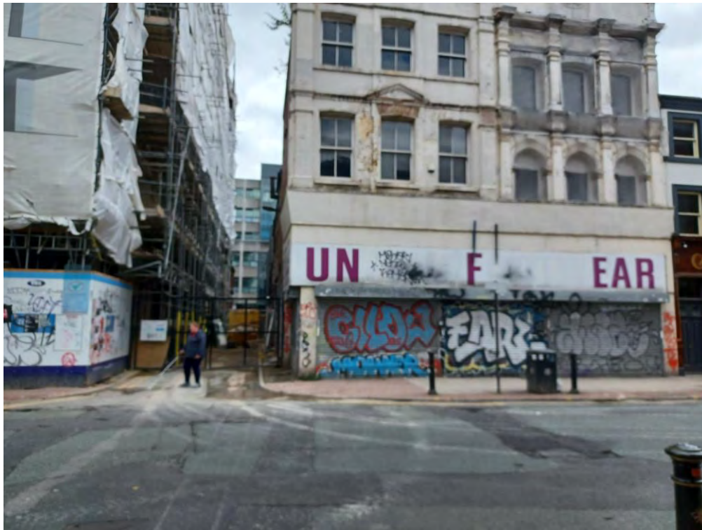
Photo 1: Photo taken at the north corner looking south east across site.
