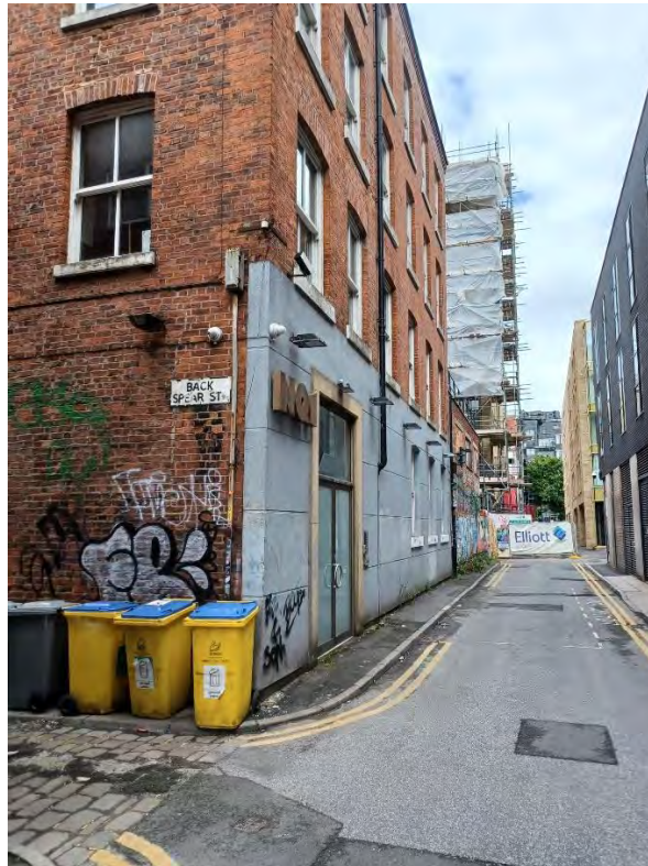
Photo 6: Photo taken at the south corner looking North across site.
