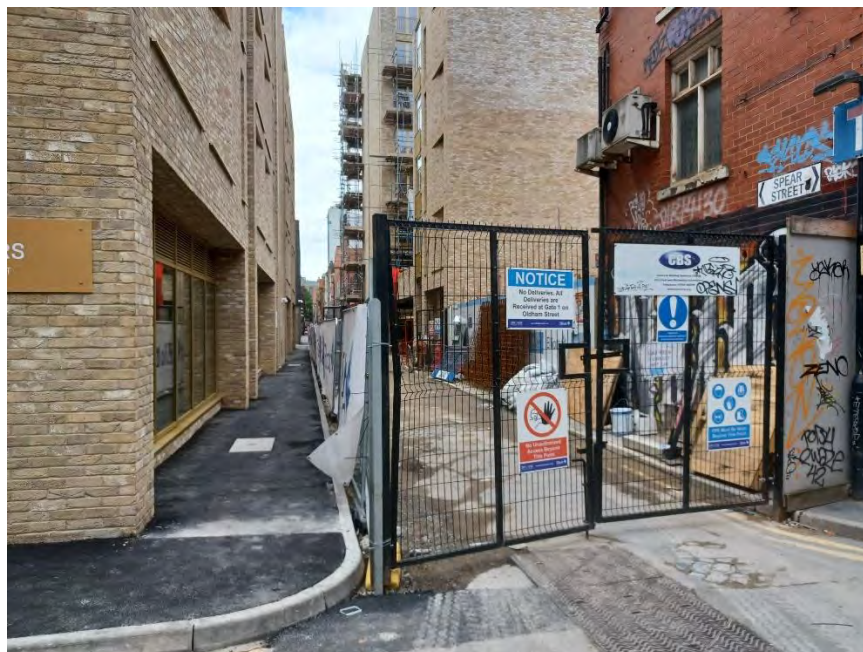
Photo 4: Photo taken east access road looking south west across site.
