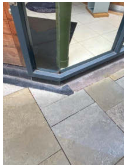
10. Continuation of tarmac infill
