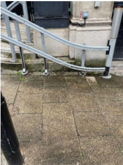
21. Stair lift condition
