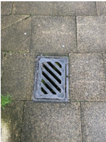
27. Clear drainage inspection chamber
