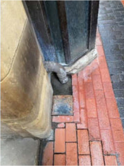
19. New installation of bricks and chipped concrete upstand
