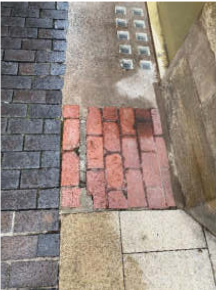
26. Concrete infill between feature bricks.
