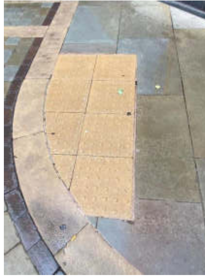
25. Missing mortar around pedestrian crossing
