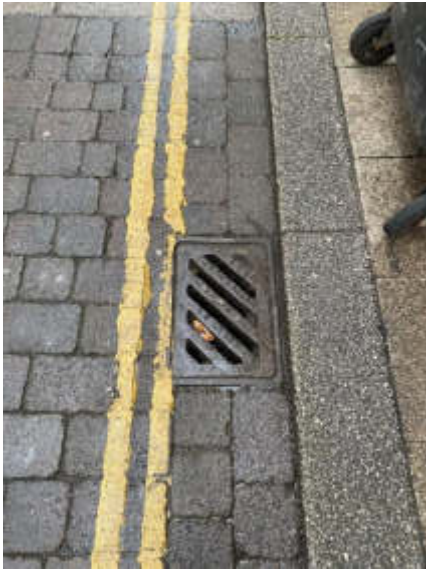
7. Partially blocked drainage inspection chamber
