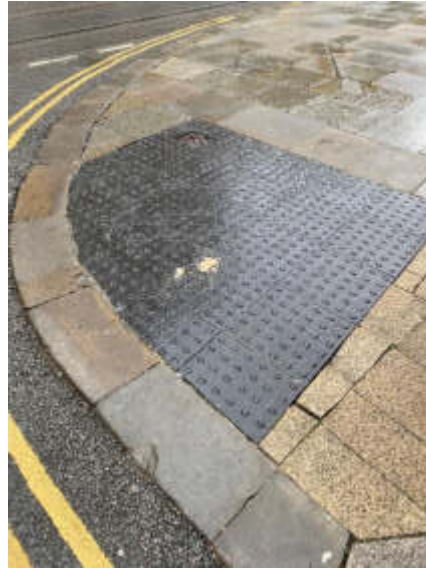
20. Pedestrian crossing condition
