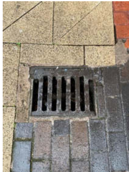
22. Empty drainage inspection chamber
