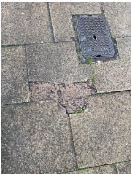
23. Concrete infill to damaged tiles
