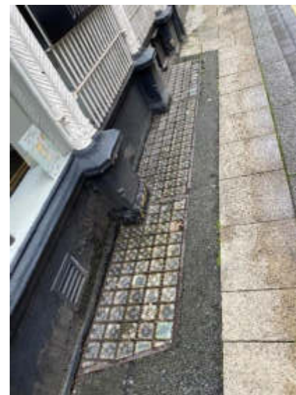
6. Overall condition of glass tiles
