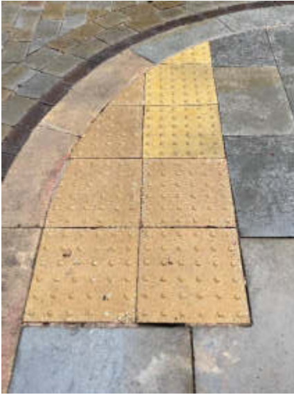
25. Missing mortar around pedestrian crossing
