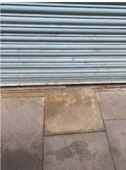
5. Raised section and concrete infill into paving
