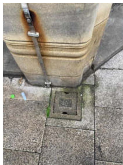
6. Earth core chamber
