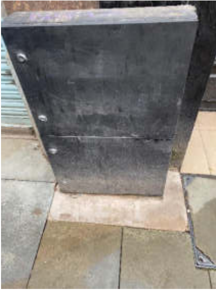
1. Service box identified, no current damage seen.
