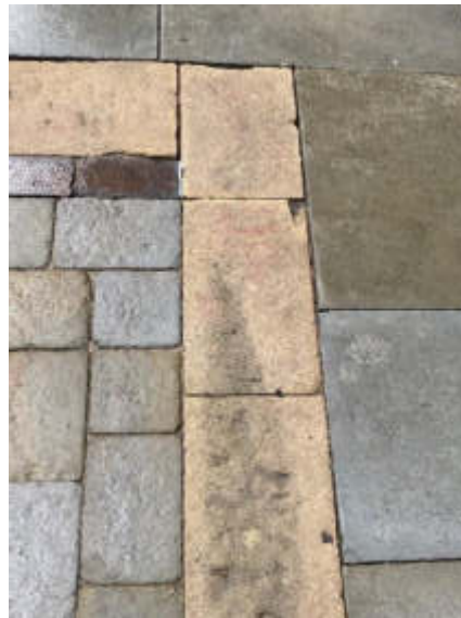
43. Damage to edge paving, Evidence of pooling due to vegetation growth
