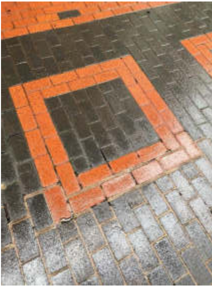
7. Replacement mortar – change in colour
