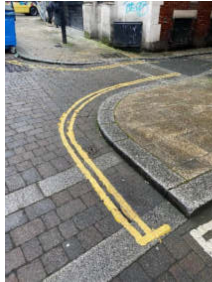
32. Repainted double yellow lines
