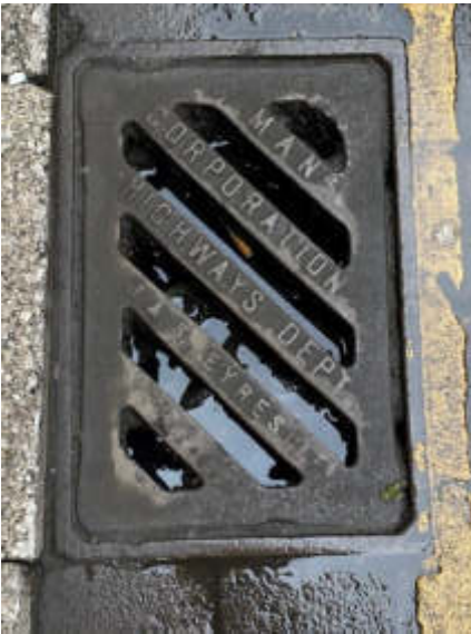
7. Blocked drainage inspection chamber
