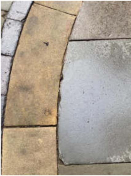
31. Chipping to paving stone
