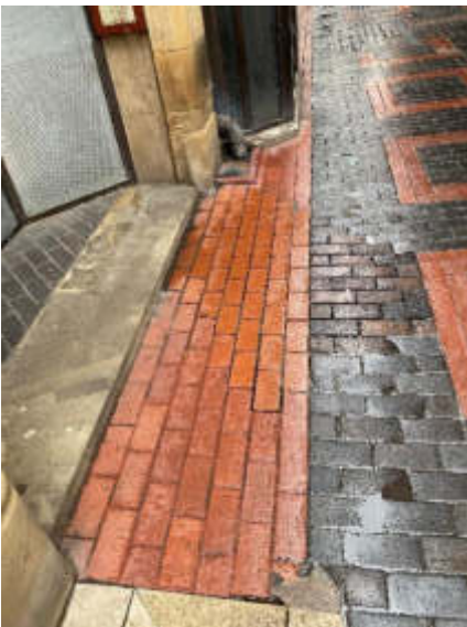
21. Change in brick type / new bricks Concrete infill to end of red bricks
