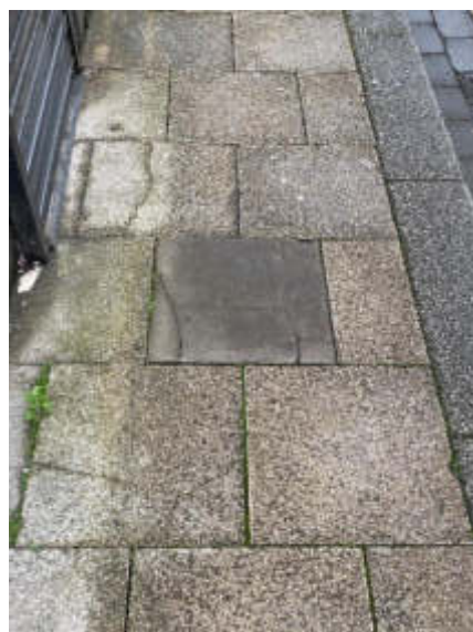
28. Replacement tile and multiple cracks
