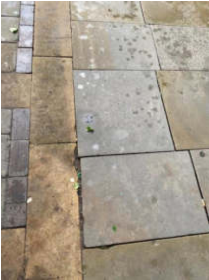
43. Damage to edge paving, Evidence of pooling due to vegetation growth
