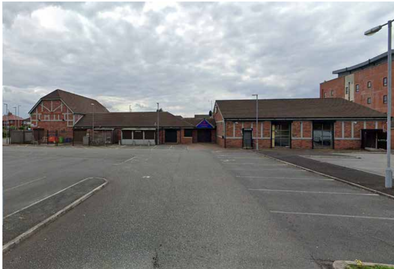
FIG 11. REAR OF EXISTING BUILDING FROM CAR PARK
