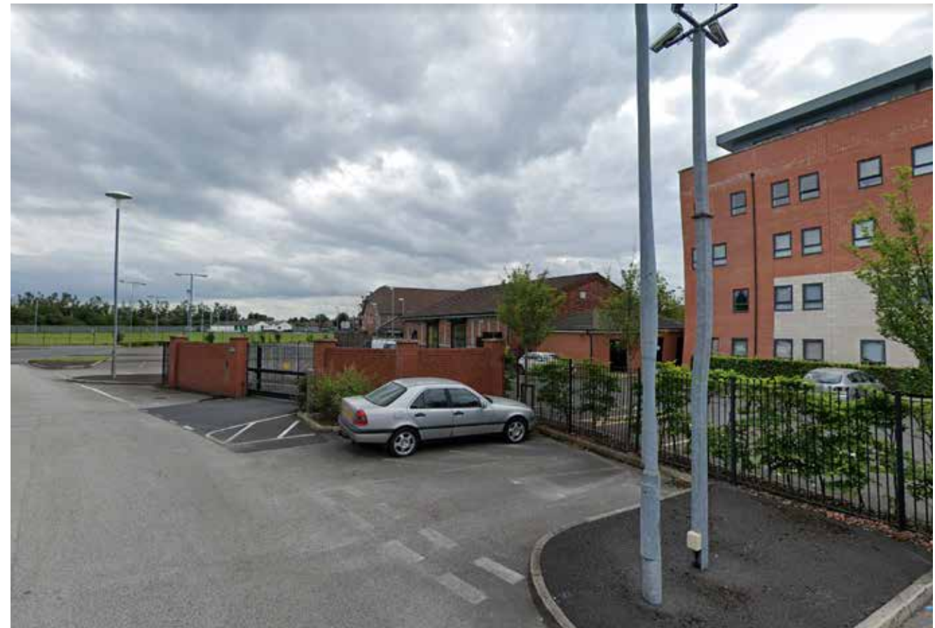
FIG 12.VIEW TOWARDS REAR OF BUILDING FROM ADJOINING CAR PARK
