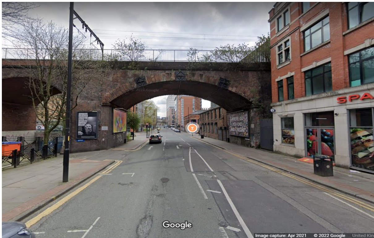
Princess Street Crossing – April 2021
