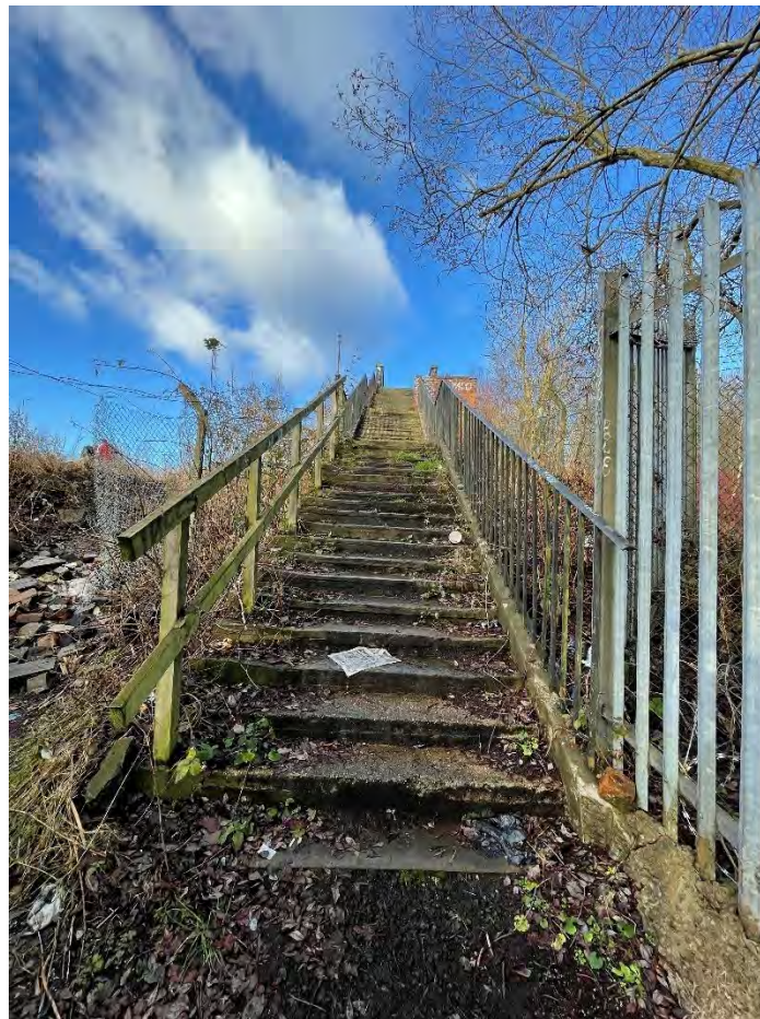
Photograph 5: Stairway at southern extent of Lowry Footbridge
