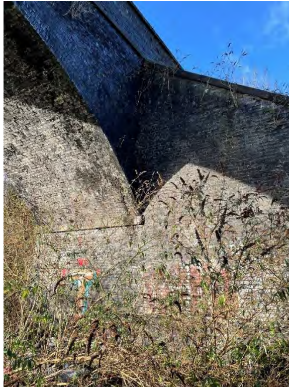
Photograph 4: Close up view of fabric of Lowry Footbridge, camera facing north
