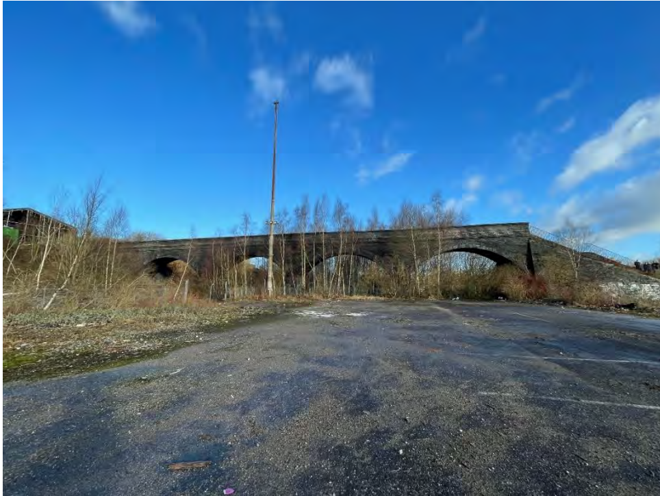
Photograph 3: View of Lowry Footbridge, camera facing northeast
