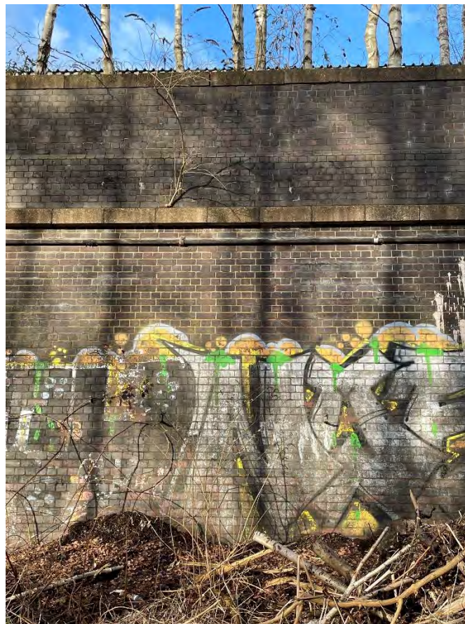
Photograph 11: Close up view of fabric of Modern retaining wall
