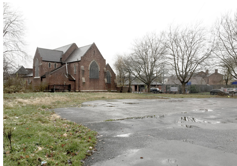
03. View facing Bacup Street
