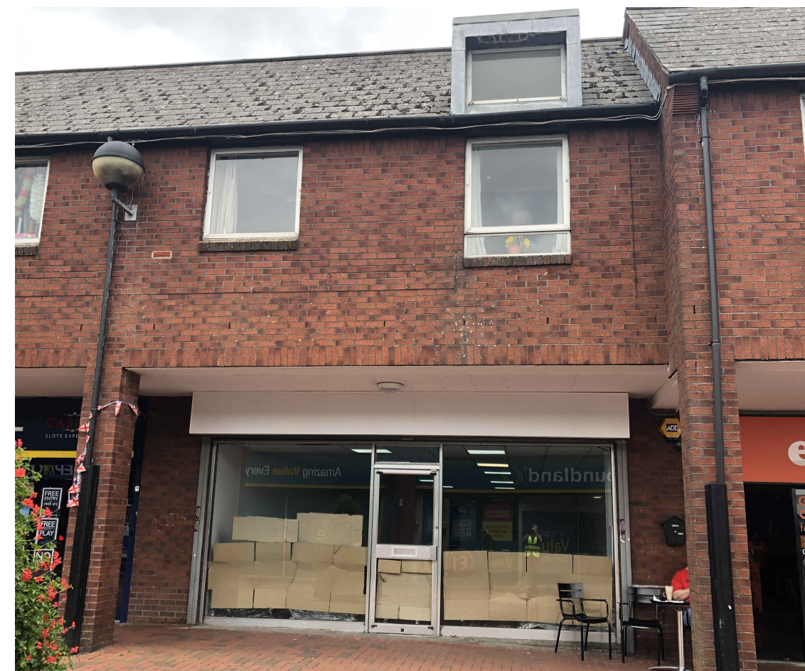
Existing Shop Front - Photo
