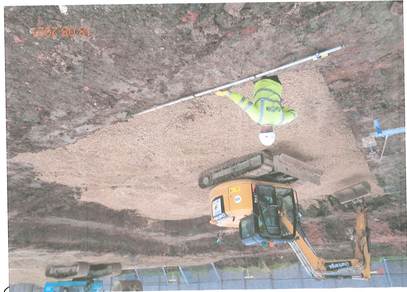
CAR PARK SITE - ATTENUATION TANK - 18.08.21 (EXCAVATION + PREP FOR TANK INSTALLATION)
