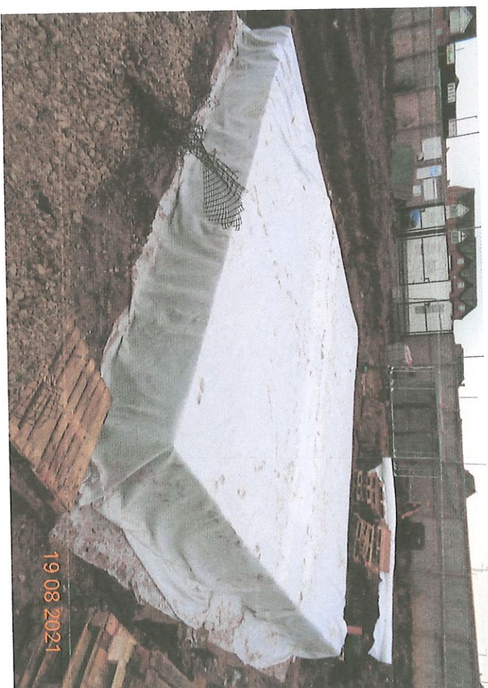
CAR PARK SITE: ATTENUATION TANK INSTALLED - 19.08.21
