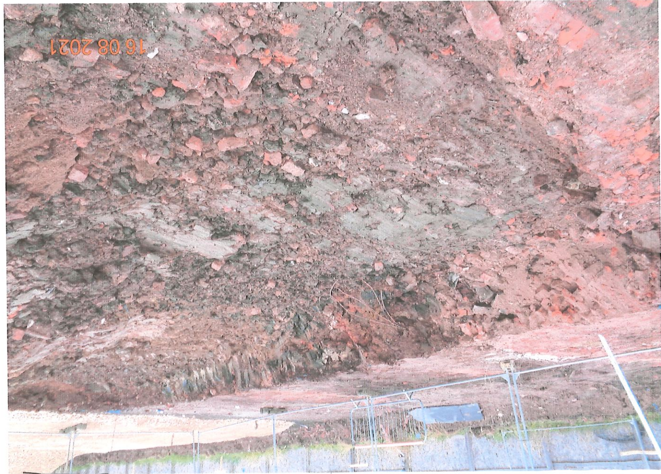
CAR PARK SITE - START EXCAVATION OF ATTENUATION TANK
