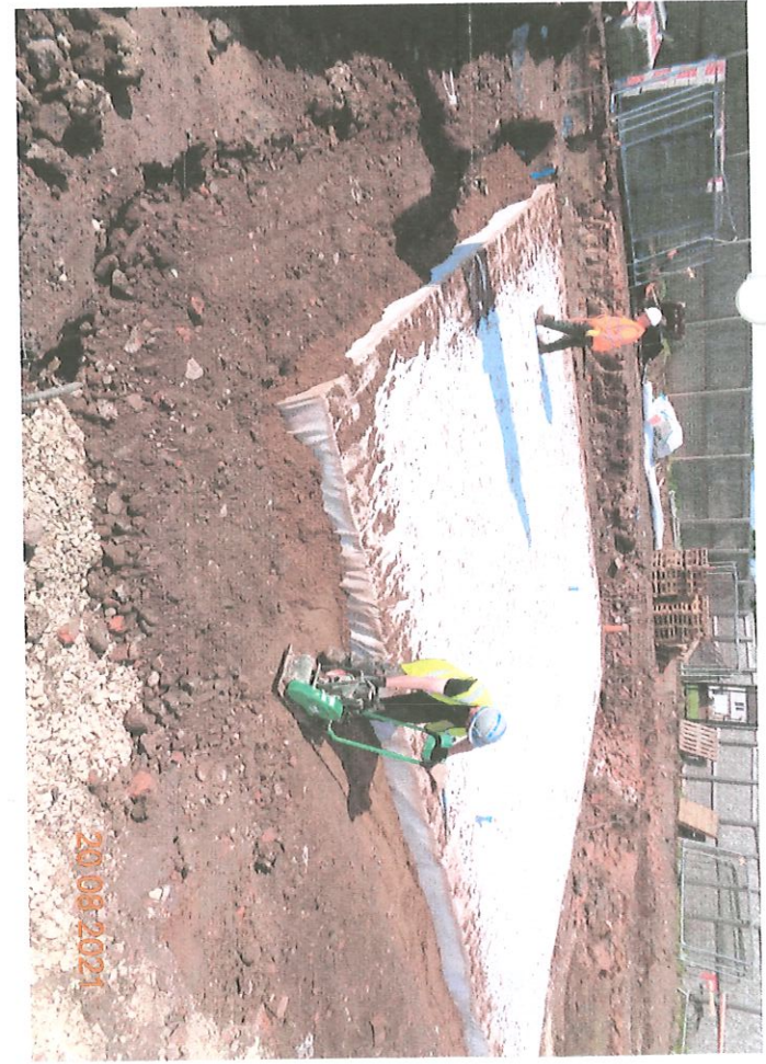
CAR PARK SITE - BACKFILLING ATTENUATION TANK - (20.08.21)
