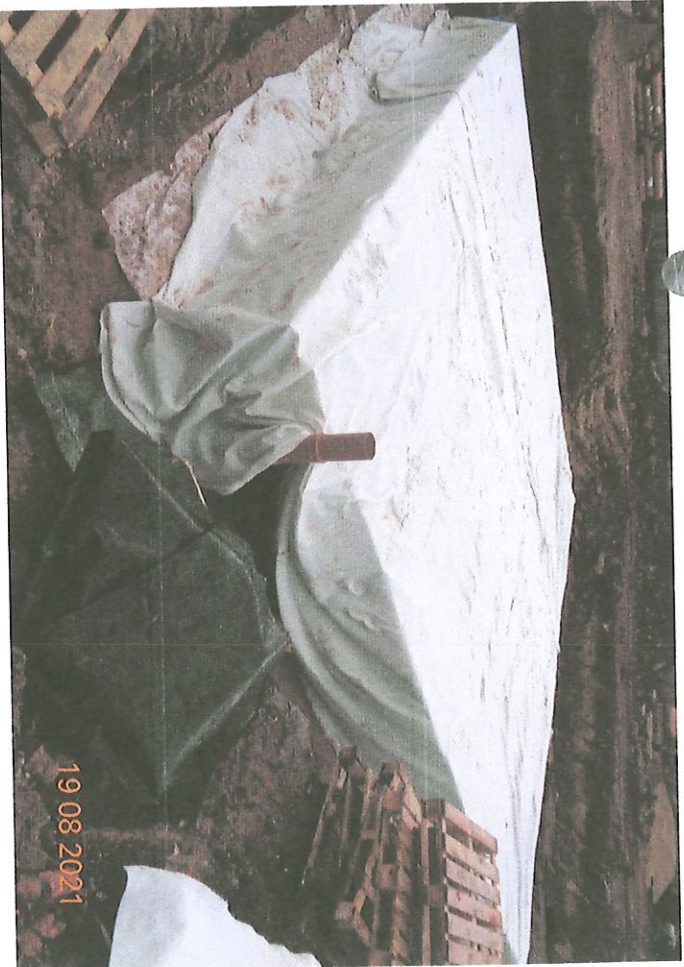
CAR PARK SITE: ATTENUATION TANK INSTALLED - 19.08.21
