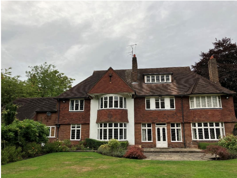
PLATE 3 VERTICAL DECORATIVE TILES AND SEALED SOFTFIT BOX ON THE BUILDING
