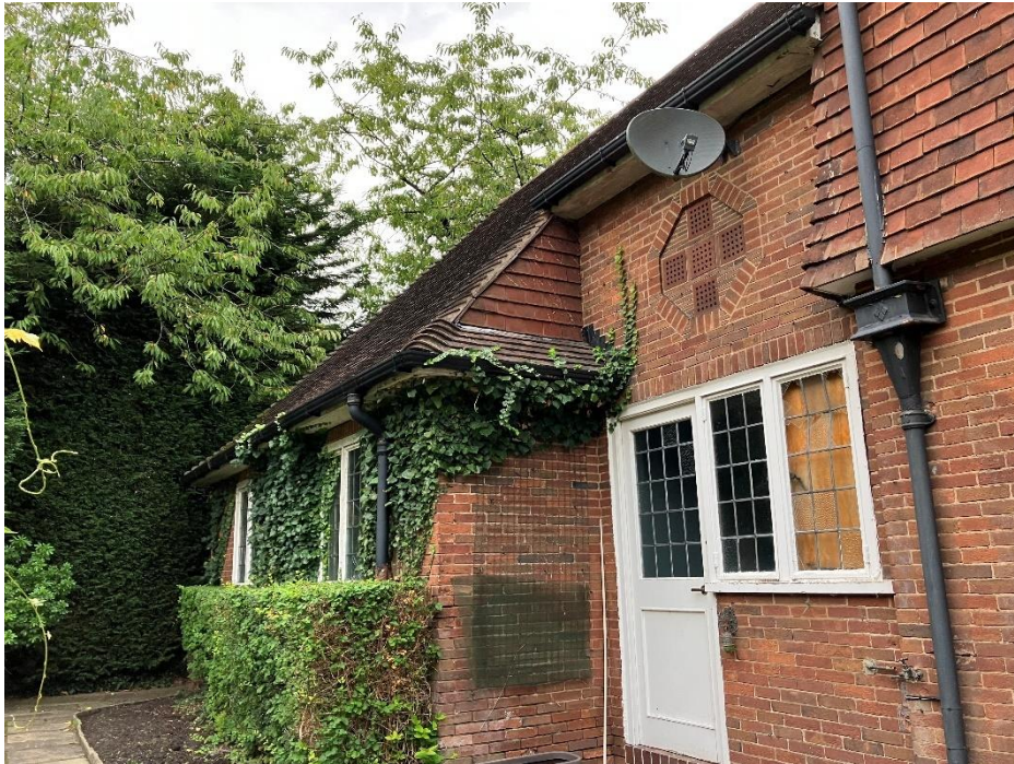
PLATE 4 VERTICAL TILE SLATES, WINDOW SEALS, AND BRICKWORK ON THE BUILDING
