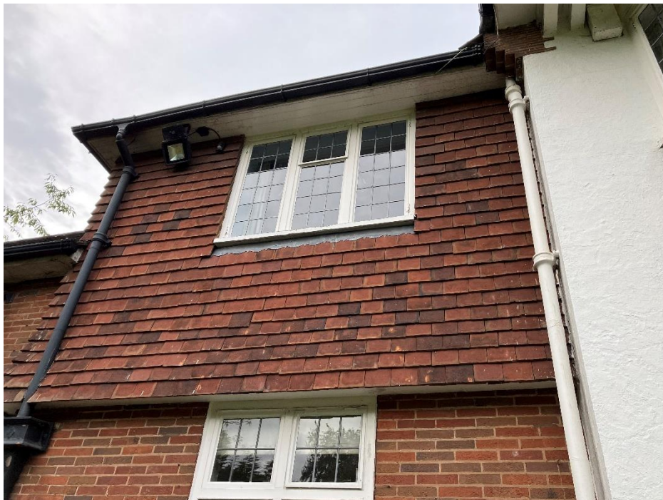
PLATE 3 VERTICAL DECORATIVE TILES AND SEALED SOFTFIT BOX ON THE BUILDING
