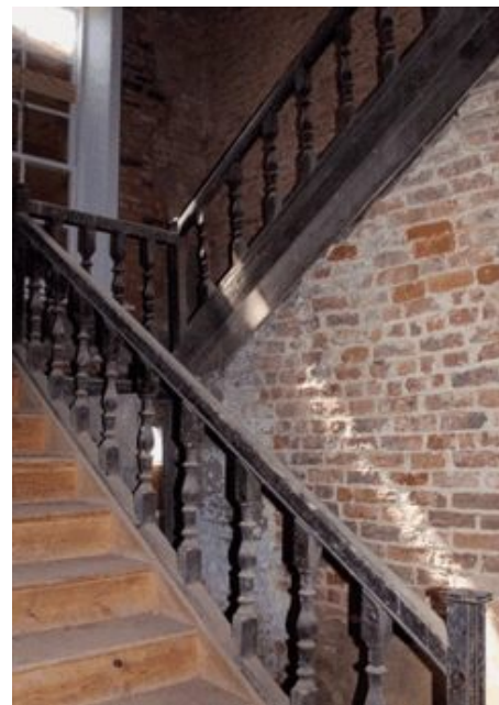
Plate 39 Stair in Room 0/21
