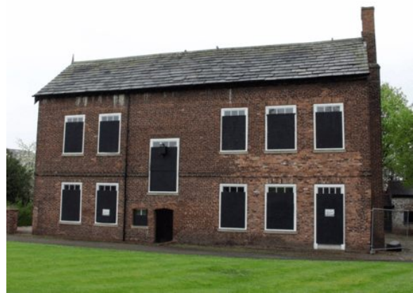
Plate 36 South elevation of the south wing
