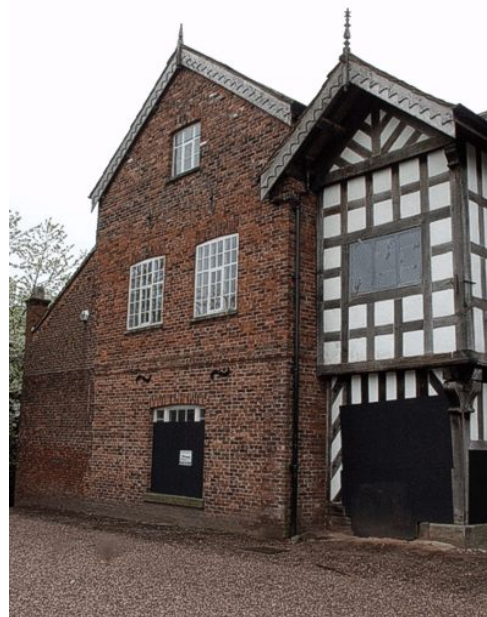
Plate 24 The brick facade of the north wing
