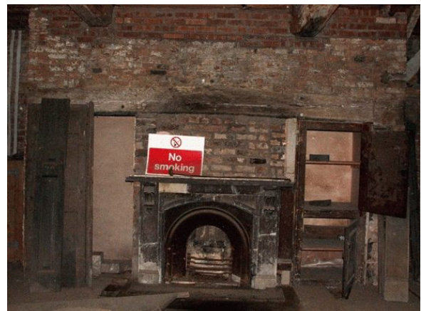
Plate 28 Fireplace in Room 0/15
