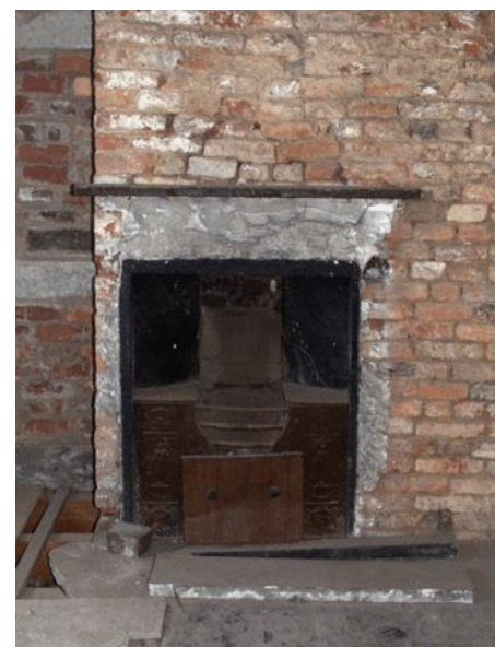
Plate 33 Fireplace in the north wall of Room 1/08
