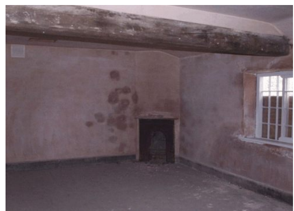
Plate 35 First-floor living accommodation in the northern extension (Room 1/04)
