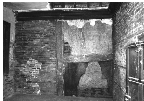
Plate 30 Timber-framing revealed by restoration
