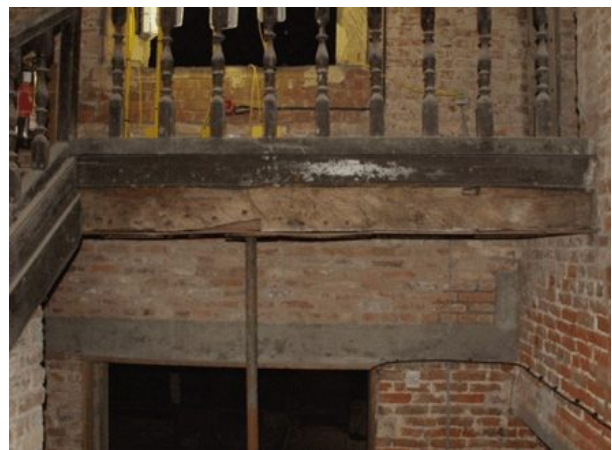
Plate 6 Re-used timber in the stair of Room 0/21
