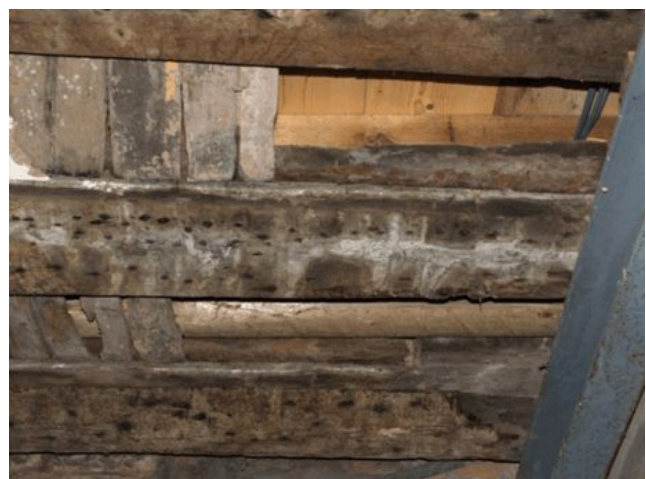
Plate 5 Elaborate ceiling construction in Room 0/09
