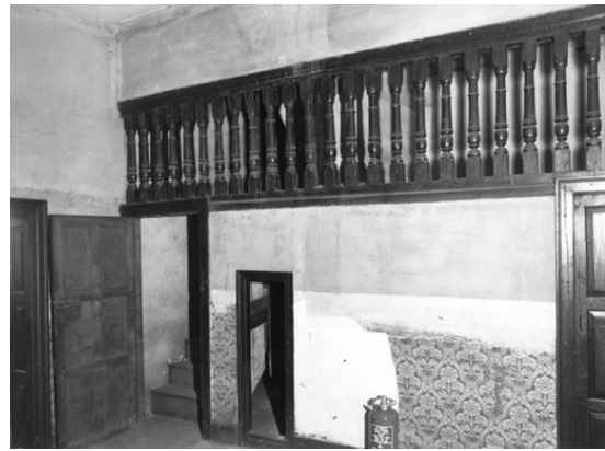
Plate 31 Photograph taken in the 1960s, showing forming subdivision of Rooms 1/05 and 1/06
