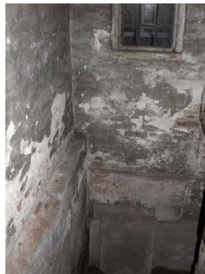
Plate 37 Inserted stair down to basement
