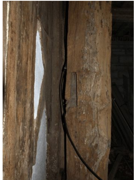
Plate 4 Empty mortice in Room 0/15
