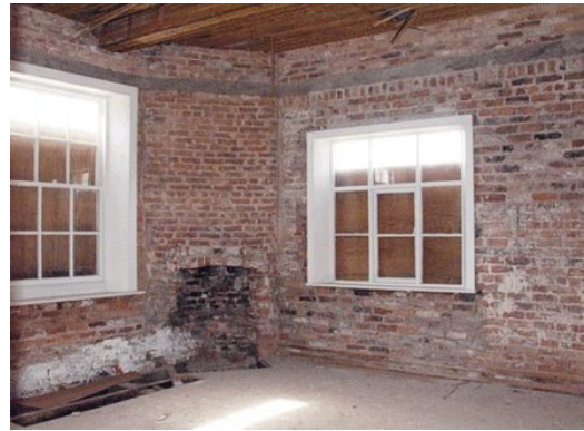
Plate 40 Room 0/23 looking southwest
