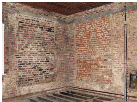
Plate 42 Room 1/12 looking northwest
