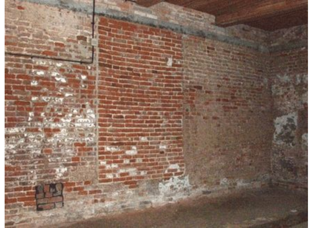
Plate 38 Blocked opening in the north elevation of Room 0/18
