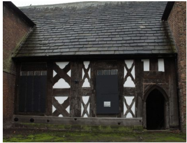
Plate 3 East external elevation showing massive plank construction
