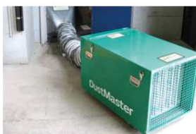
DUSTEX DUSTMASTER Self - contained dust extraction/filtration unit
