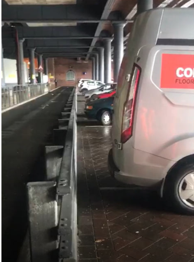
PHOTO 03 LOCATION OF GENERAL EV CHARGING BAYS
