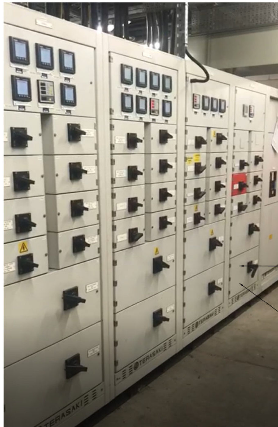
PHOTO 01 LOCATION OF EXISTING LV PANEL (MSB01-01)
